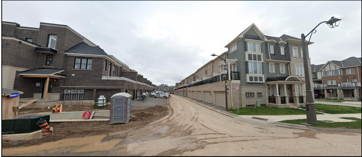
Figure 8: Street-view of Lane 166 ( garages without driveways on the right )
