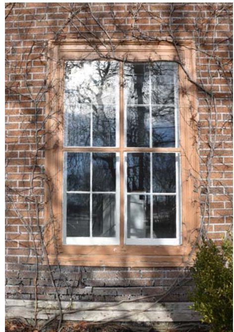
Interior and exterior views of the c.1850s first floor casement windows. The exterior storms were a later addition. Photo credit: Town of Oakville staff, 2018.
