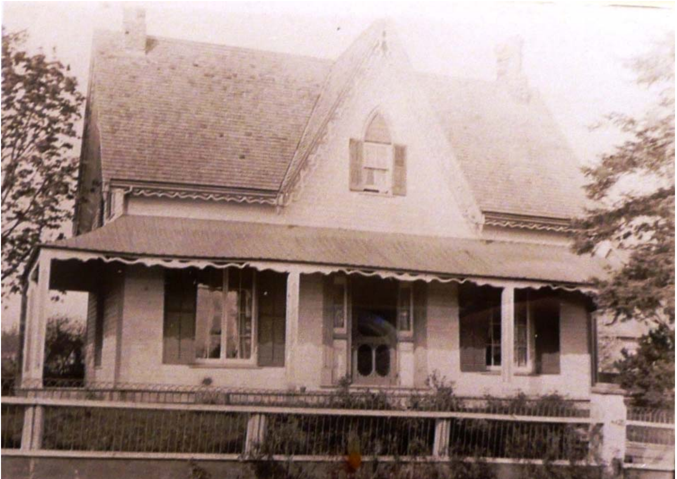
Postcard photo of the house from c.1904 showing historic features, including verandah, brick chimneys, wood siding and shutters. Photo credit: Trafalgar Township Historical Society
