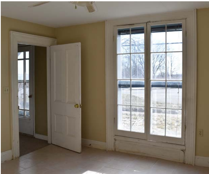
Interior and exterior views of the c.1850s first floor casement windows. The exterior storms were a later addition. Photo credit: Town of Oakville staff, 2018.
