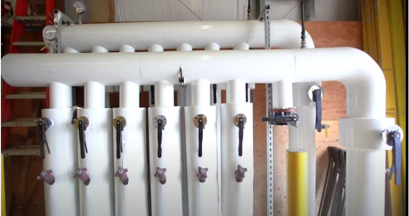
Picture 1: Blackstone Project – Conestoga College – 250-ton geothermal ground-source heat pump system
