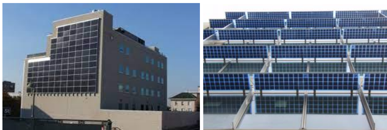
Figure 3: Example of BAPV – the PV is mounted onto the wall
