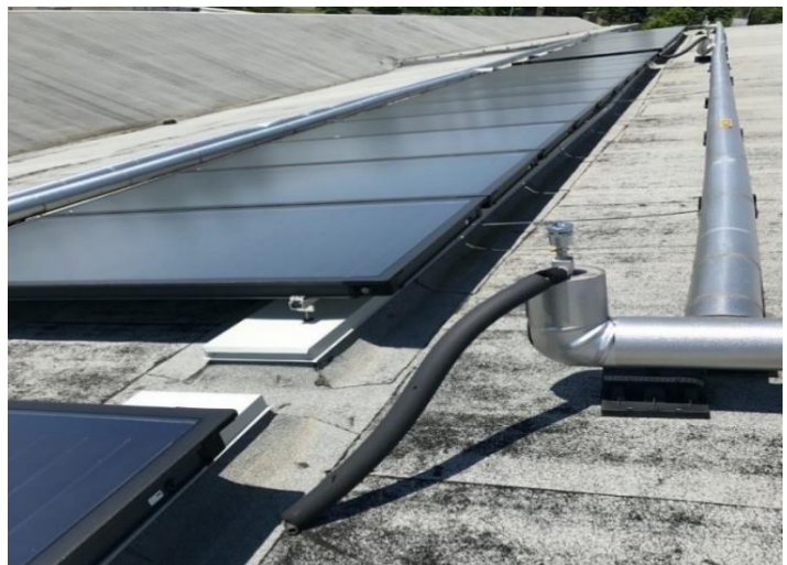
(Source: Elgin West Community Centre, Richmond Hill) Figure 22: Typical, low angle, solar panel array connection
