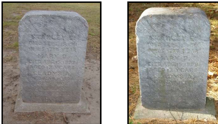
Figure 42: Stanley, Mary and Gladys Adams Vermont marble headstone immediately after restoration (November 2017) and four years later (November 2021)
