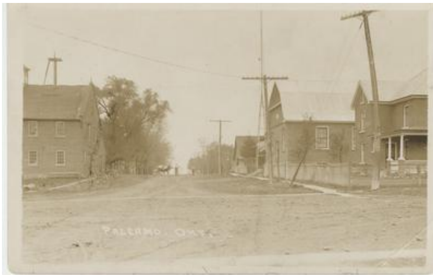
Figure 17: Postcard of Palermo looking south along Bronte Road from Dundas Street. The Lawrence Foundry building is on the left and the Community Hall can be seen on the right
