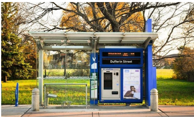
Figure 5-2: Viva Curbside Bus Stop Example
