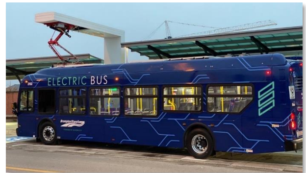
Photograph 25: Brampton Transit Electric Bus Charging
