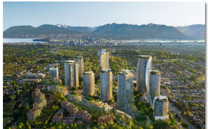
Photograph 19: Oakridge Centre Redevelopment in Vancouver
