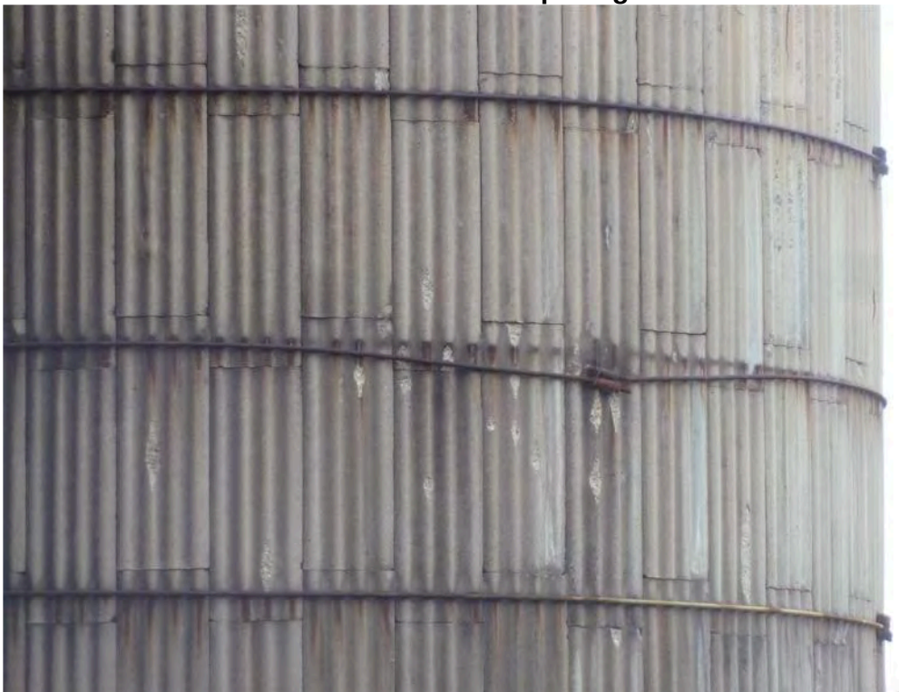
Photo 22 – East Silo – Steel Hoop Loose
