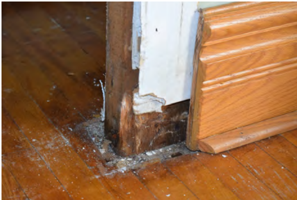
Plate 77: Close-up of water damage, October 2018
