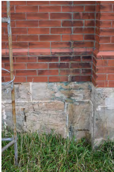
Plate 36: North elevation cracking and water stains, October 2018
