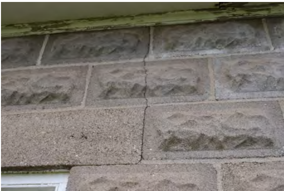
Plate 94: Concrete crack on south elevation, October 2018
