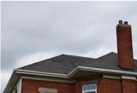
Plate 38: Weathered shingles at southwest corner of roof, October 2018
