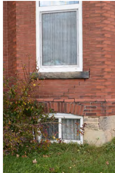
Plate 37: South elevation bay window brick cracking, October 2018
