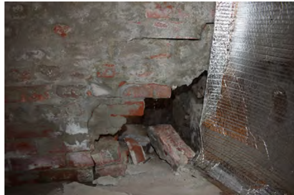
Plate 70: Hole on the interior brick wall, October 2018
