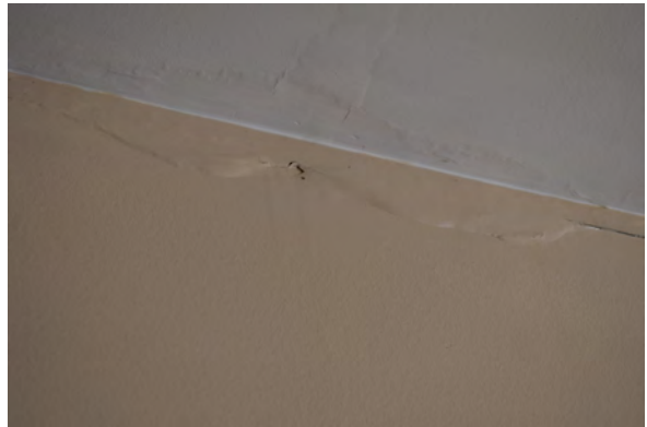
Plate 80: Water damage on bathroom wall and ceiling, October 2018
