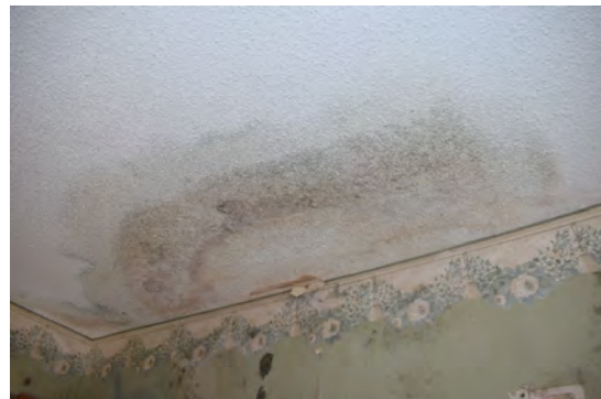
Plate 76: Close-up of water damage in bedroom, October 2018
