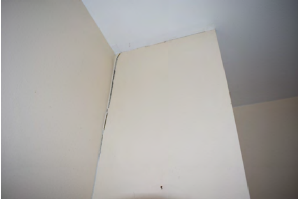
Plate 81: Crack on laundry room wall, October 2018
