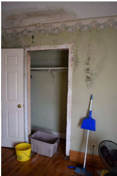
Plate 75: Water damage in bedroom, October 2018
