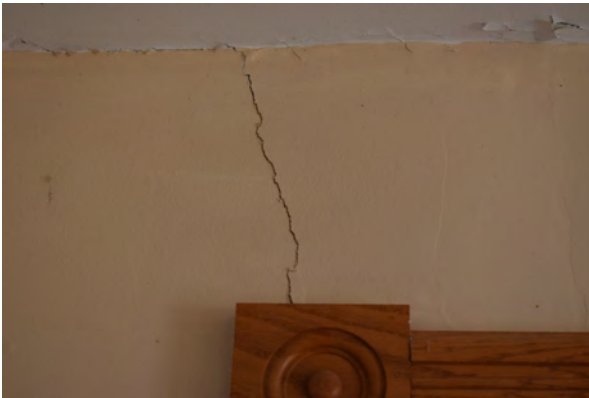
Plate 79: Cracking above bathroom window, October 2018
