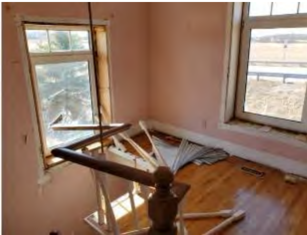
Plate 83: Interior trim removal and railing damage. Photo courtesy of Bell Mobility, September 2020
