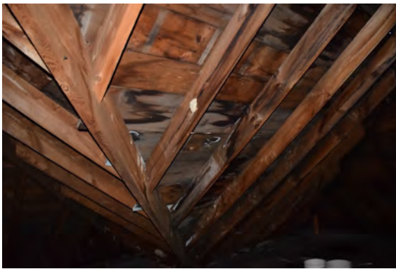
Plate 86: Water damage in attic looking southwest, October 2018
