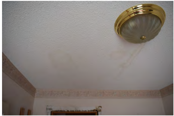
Plate 78: Water stains on bedroom ceiling, October 2018
