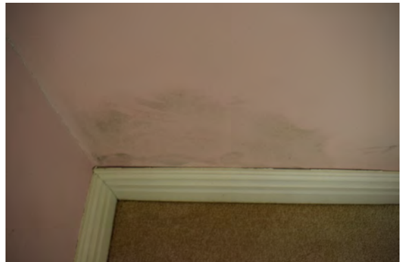
Plate 51: Close-up of water damage and mould on staircase landing, October 2018
