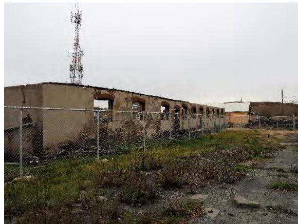
Plate 21: Barn window and door openings following fire damage, November 2020
