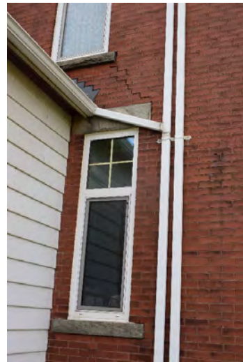
Plate 35: East elevation brick cracking above window, October 2018
