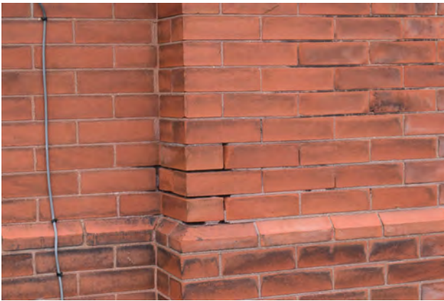
Plate 34: South elevation evidence of mortar receding and falling from joints, October 2018
