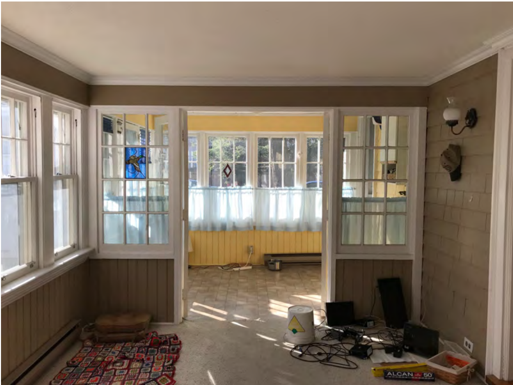
SUNROOM – original wood windows & doors – original wood shingle on the cottage is visible inside the sunroom
