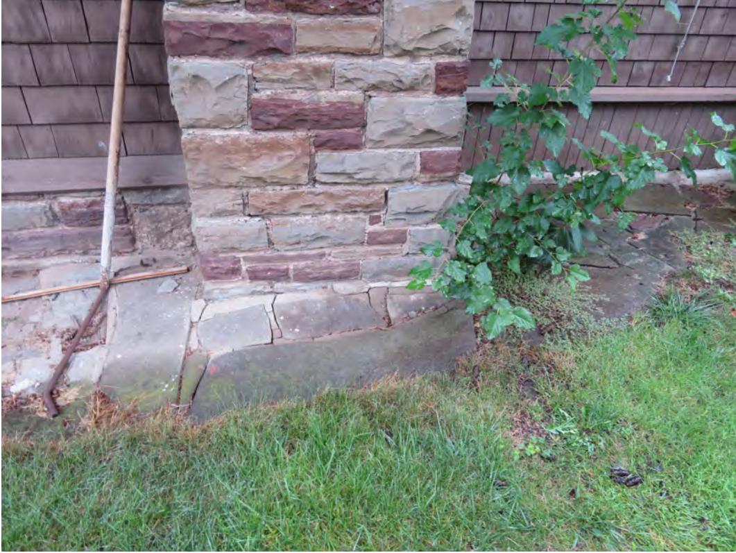
Flagstone paving – loose and missing mortar at the base of the masonry pier
