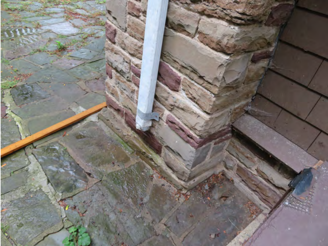
Flagstone paving – quarry cut Credit Valley sandstone
