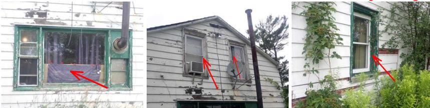
3. **Siding** Siding - Siding is falling apart allowing water to penetrate the in behind structure. This has caused the structure to rot and shift over the years, which has compromised the overall stability of the home. This results in an unsafe place to live.
