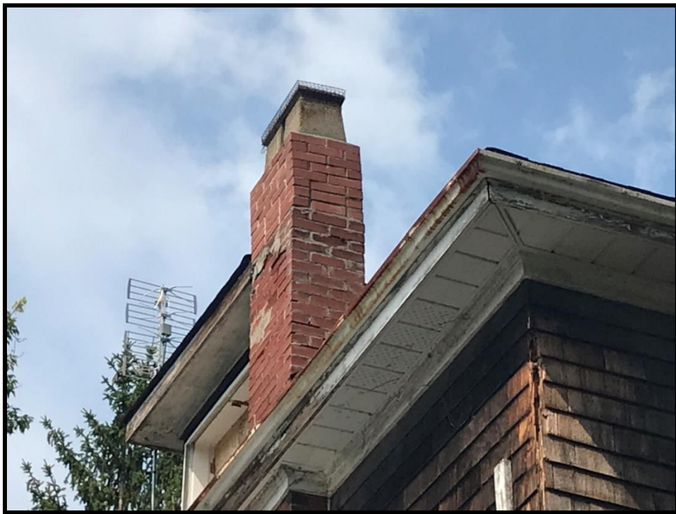
Image 6: Exterior of 164 Douglas Avenue – Chimney Deterioration (Photo taken on July 6, 2021; Facing Northwest)
