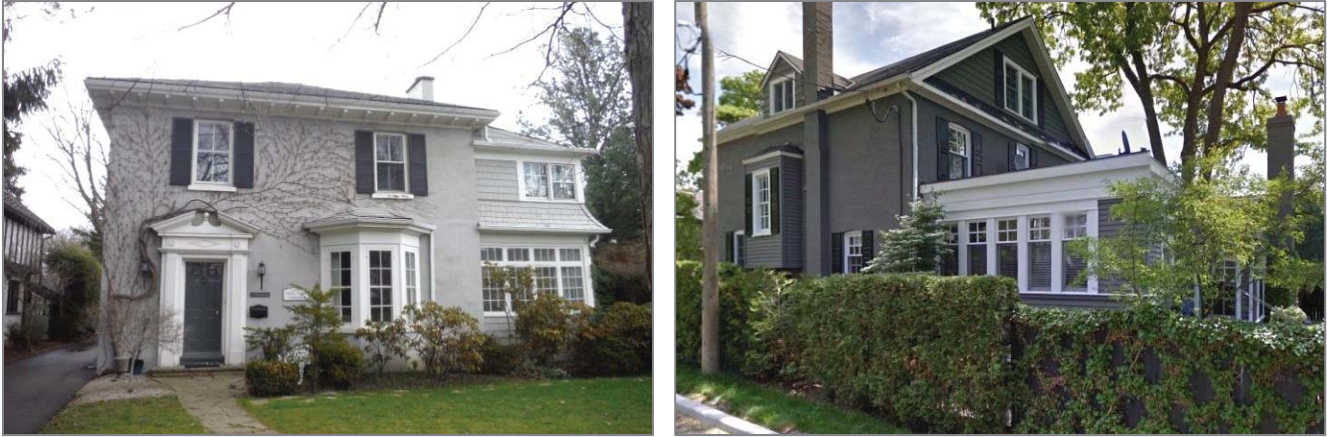
Figure 14: 75 Second St. - an 1850s house with a compatible early 20th century two-storey addition set back to the side of the main elevation (left); 56 Second St. – a 1914 house with a compatible 2002 one-storey addition at the rear of the main structure (viewed from side elevation on Union St.) (right).
