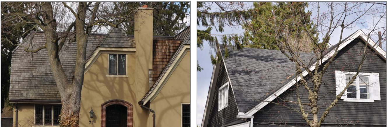
Figure 3: Cedar shingle roofing on 71 First St. (left); asphalt shingle roofing on 48 First St. (right).
