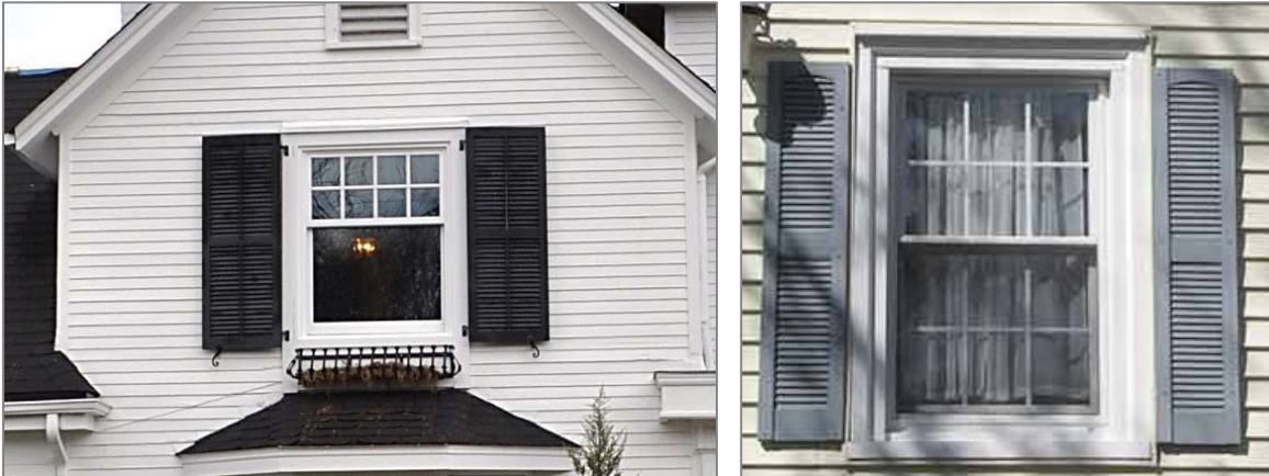
Figure 7: Appropriately-sized shutters on 66 Second St., (left); inappropriately small shutters on a building not located in the District (right) (source: http://www.oldhouseguy.com/shutters/ ).
