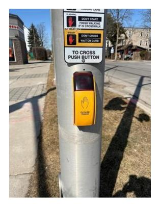
Figure 29: Pushbutton Missing Tactile Directional Arrow
