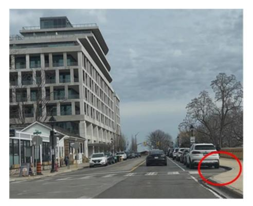
Figure 30: Crosswalk with curb ramp missing
