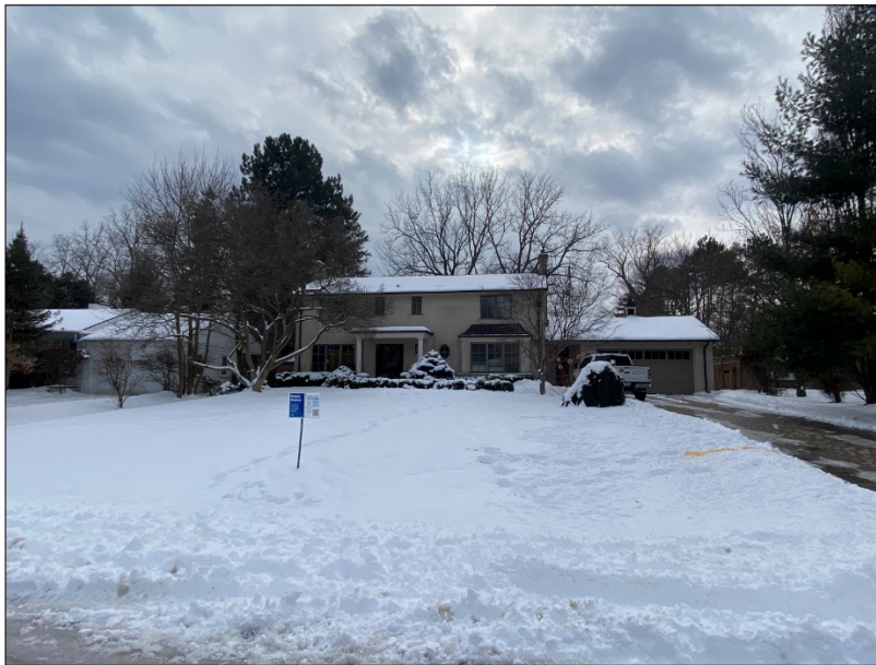
Existing Dwelling – 190 Donessle Drive (Photo taken February 11, 2025)
