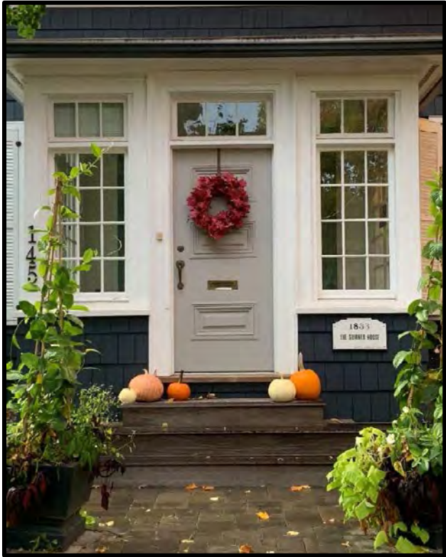
Figure 25: 145 William Street – Main entrance wood door facing street
