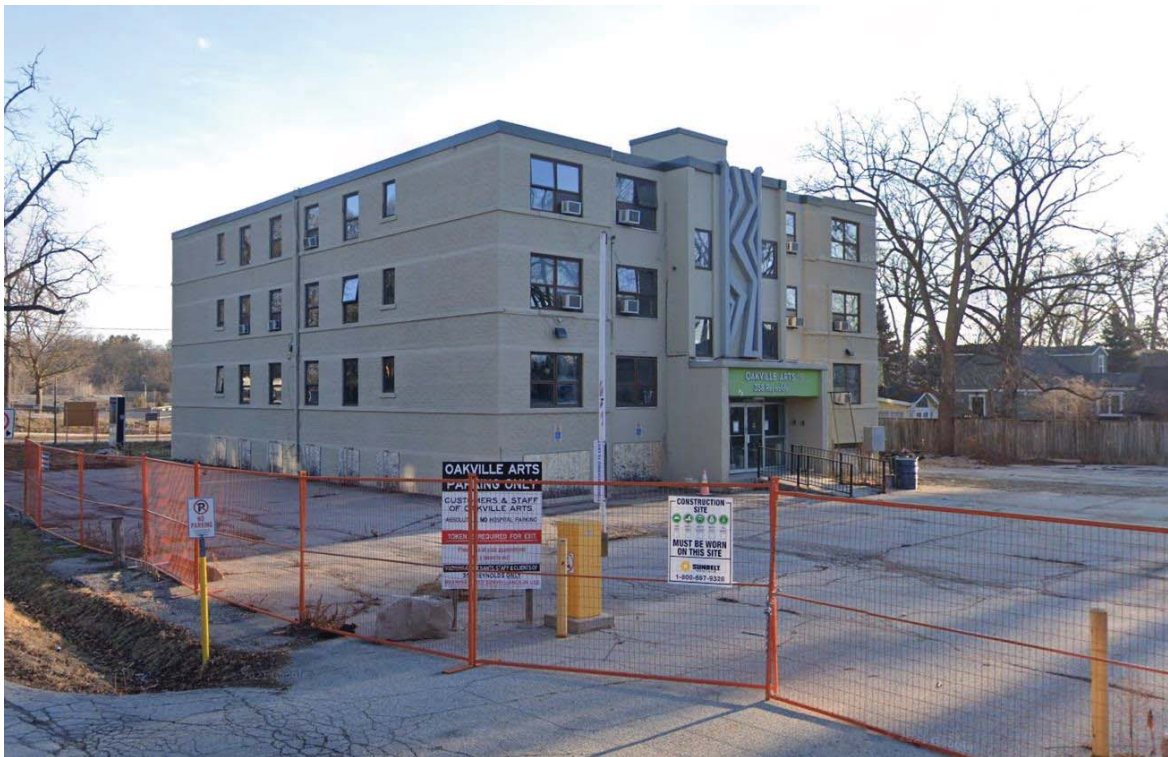
4.1.5.1.C – Existing Rear (Southwest) Elevation
