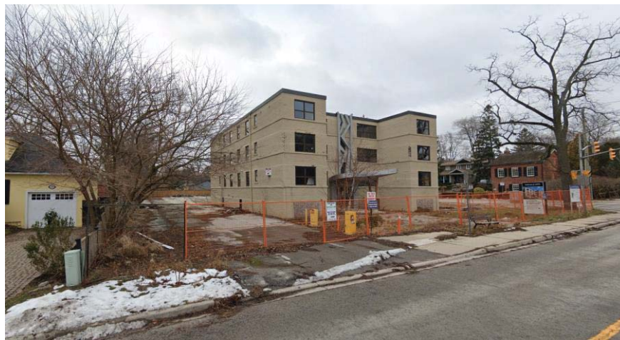
4.1.4.A - Driveway Access – Reynolds St.
