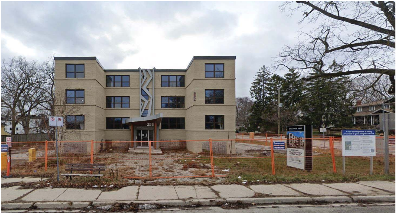
4.1.5.1.A - Existing Northeast (Front) Elevation
