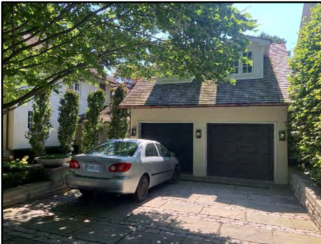
Figure 38: 66 Dunn Street – Attached 1 ½ storey garage with appearance of detachment through single storey connection to main residence
