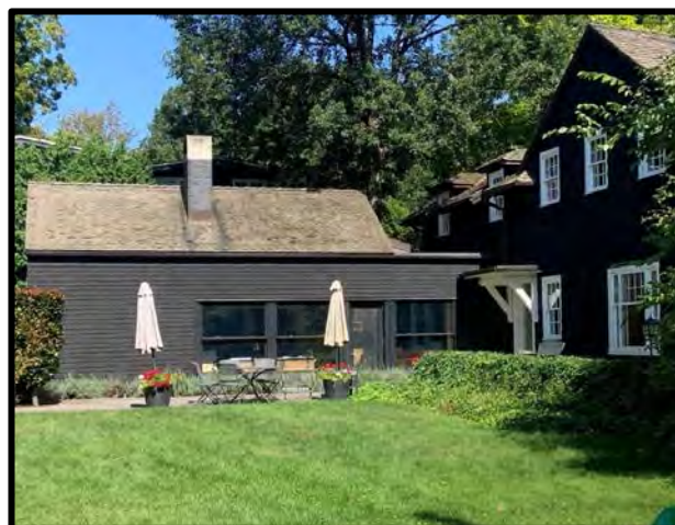
Figure 62: 308 William Street (left) – addition to rear and visible from Reynolds Street. Height of addition is lower than original, consistent horizontal wood cladding and chimney style, wood French doors in complementary style
