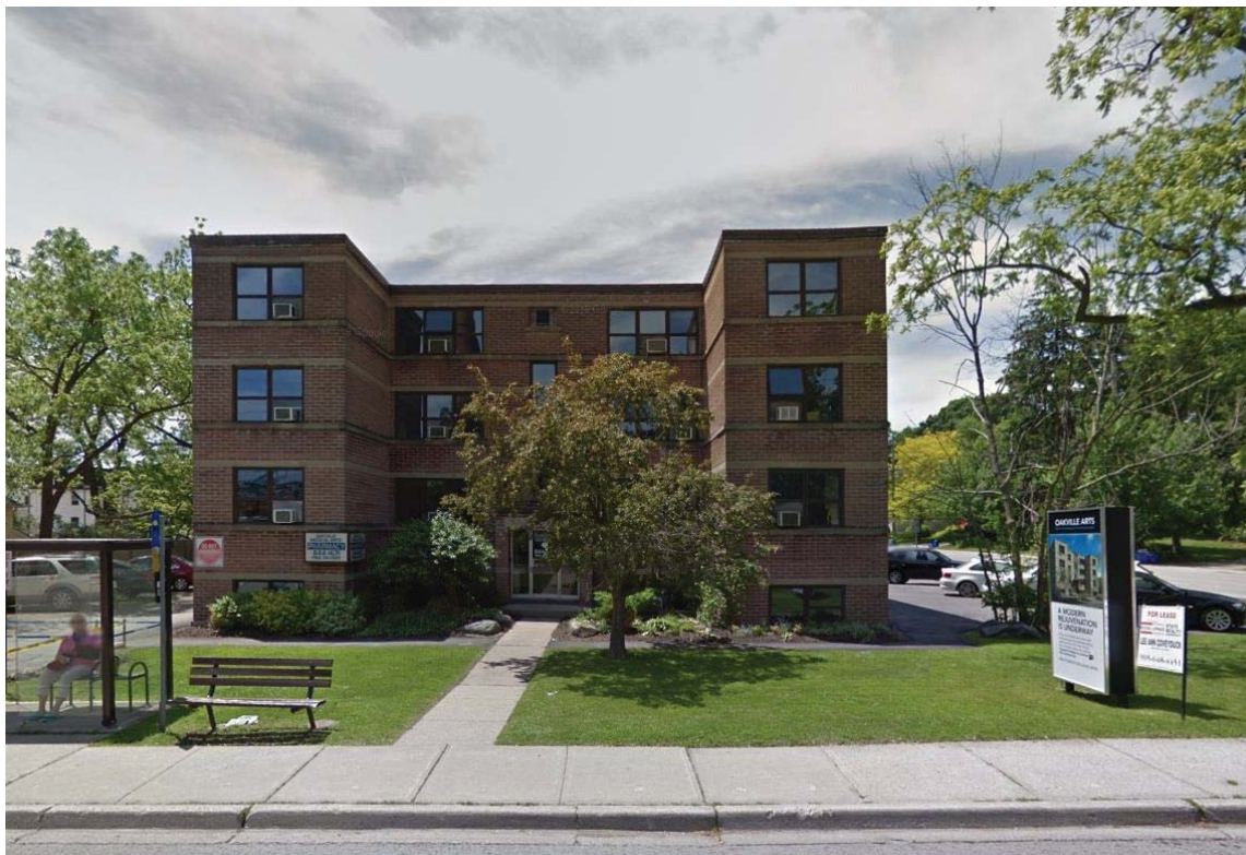
4.1.5.1.E – Existing Front (Northeast) Elevation – 2011
