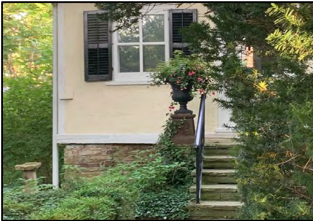
Figure 26: 115 William Street – Lakestone foundation
