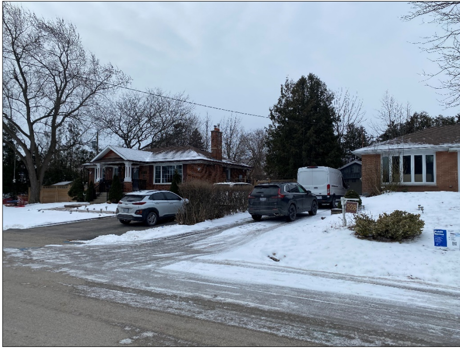
Lands to the south – 522 Weir Avenue
