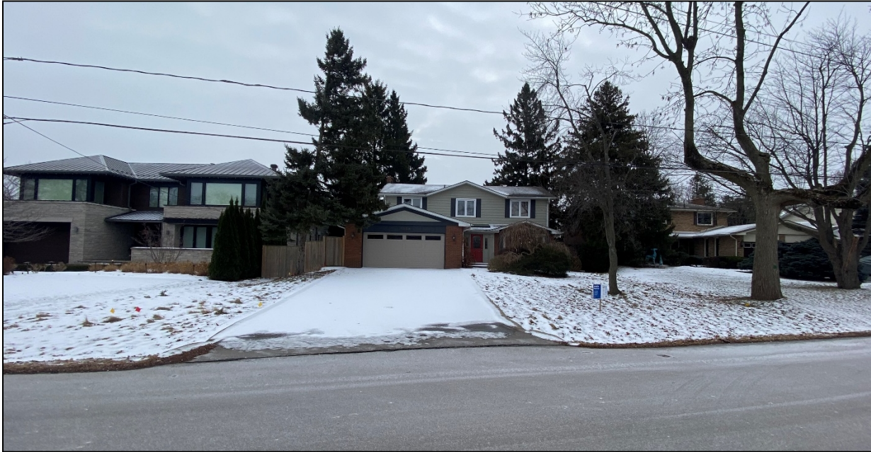
Existing dwelling located at 1574 Old Lakeshore Road
