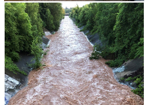
Hager-Rambo Creek Outlet at Maple Avenue – July 13, 2024
