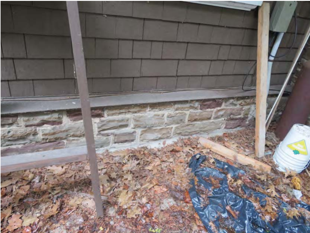
Raised stone foundation
