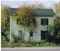
G. 3015 Dundas St., c. 1848, a Hager house, demolished 2008 (TTHS).
