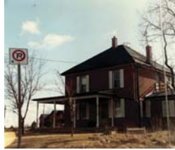
C. 2496 Bronte Rd., c. 1945, demolition date unknown.
