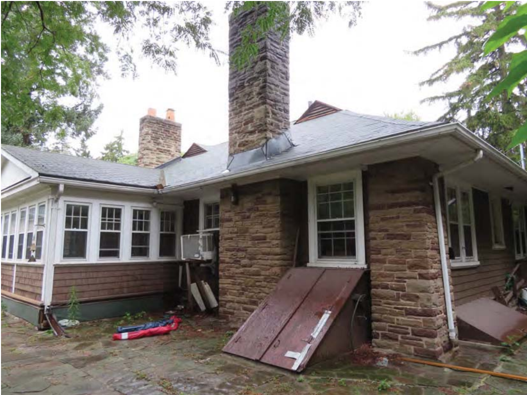
Rear elevation – sunroom – stone chimney – entrance to basement
