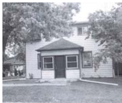
I. 2477 Bronte Road, c. 1870, demolition date unknown.
