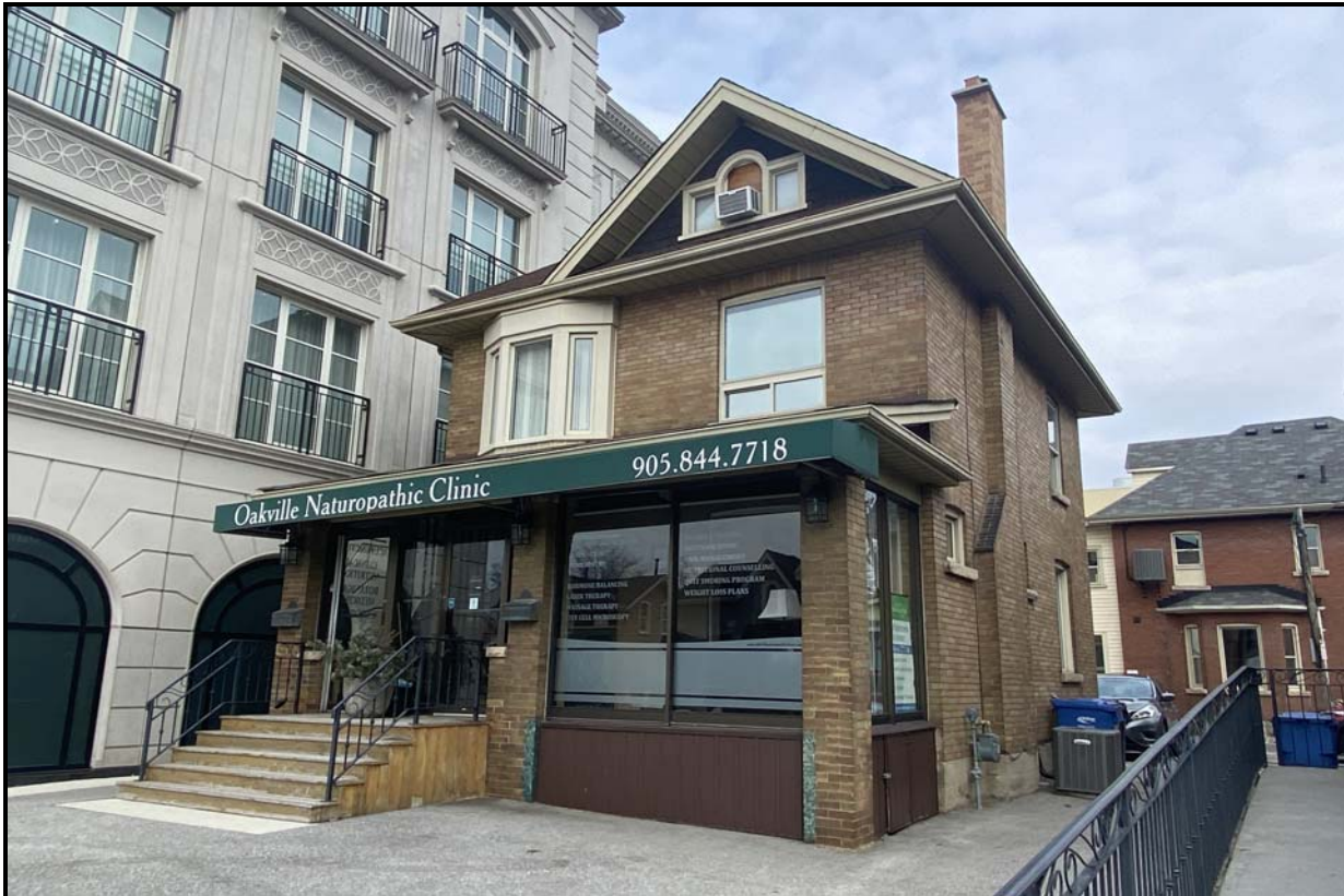
West (front) and south elevations of the building, 2024. Source: Town of Oakville Planning Services Staff
