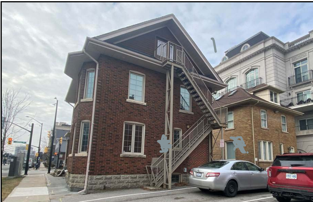
Rear elevation fenestration and view of the tower two-storey bay window on south elevation. Source: Town of Oakville Planning and Development
