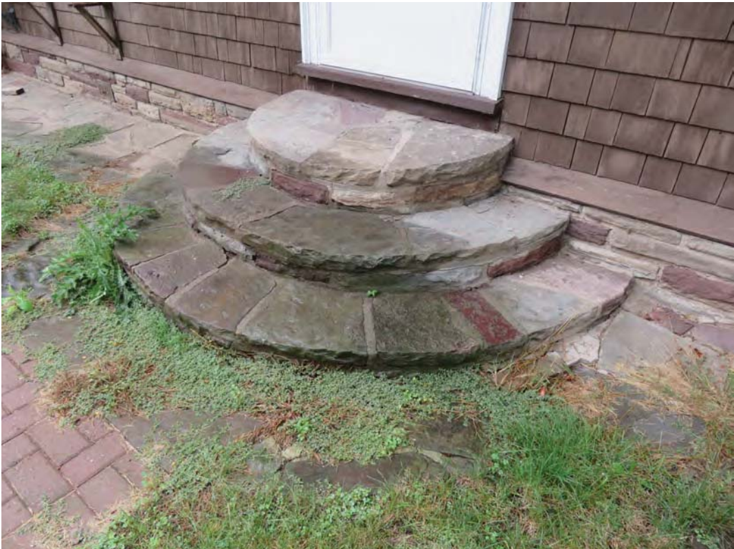
3 rounded sandstone steps at the front entrance
