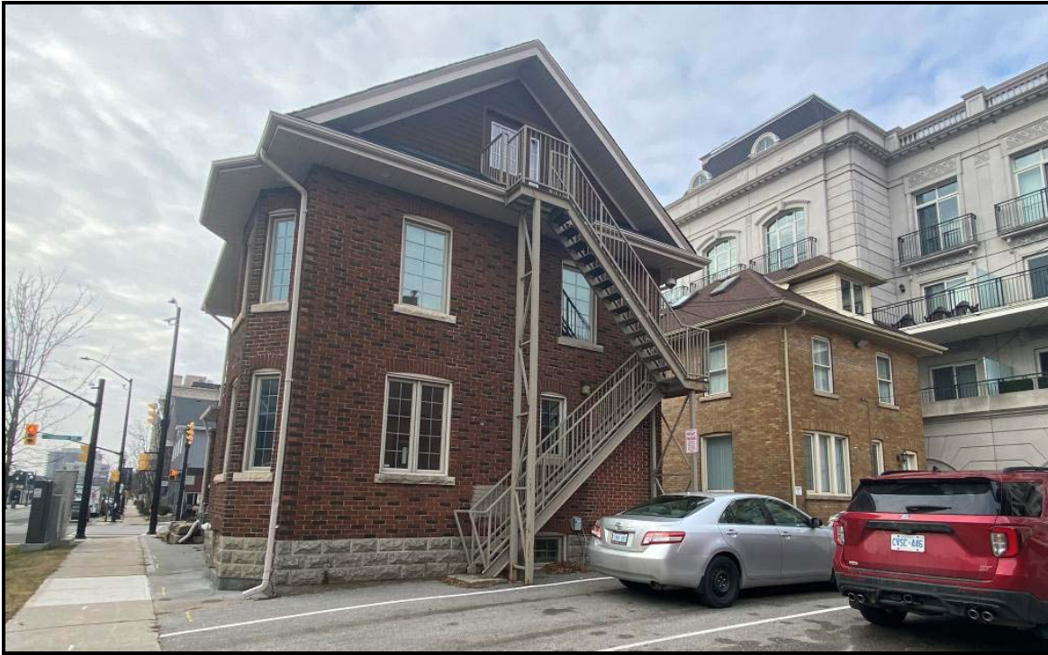
East (rear) elevation. Source: Town of Oakville Planning and Development Staff
