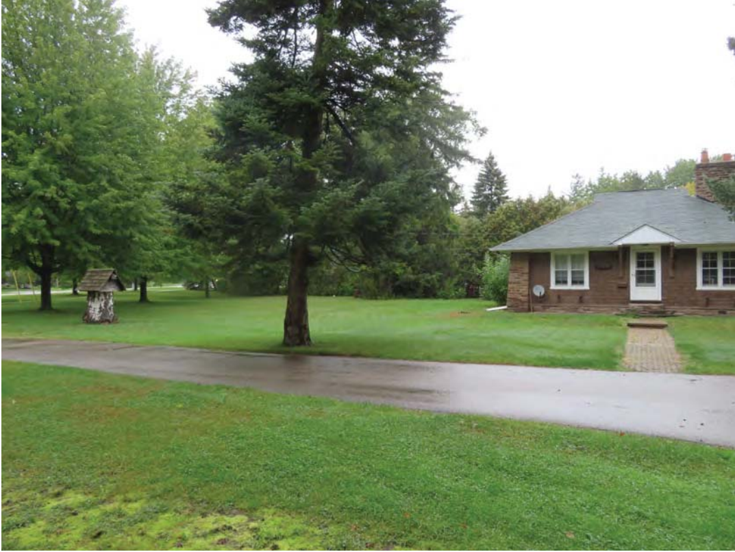
Walkway to the front door from the driveway
