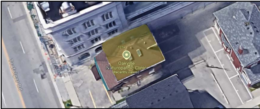
Roof shape with the central dormer at the rear. Source: Google
