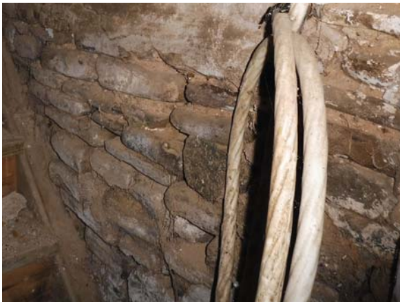
Rubble stone foundation wall in good repair (ERA, 2017).
