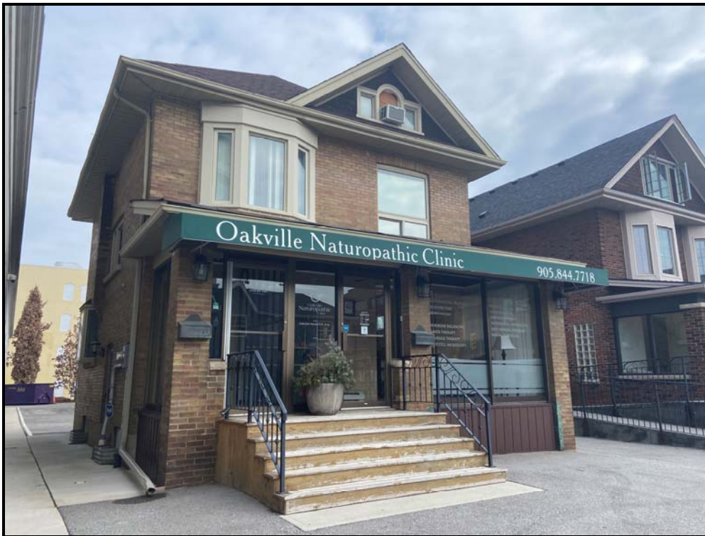
West (front) elevation of the building, 2024. Source: Town of Oakville Planning Services Staff
