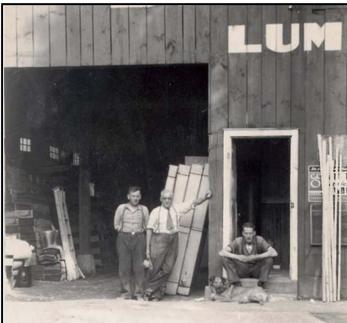
Outside the Blakelock Lumber Supplies and Planing Mill. Source: Town of Oakville files
