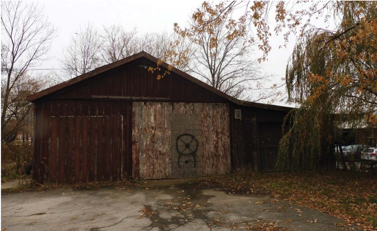
North elevation (ERA, 2017).
