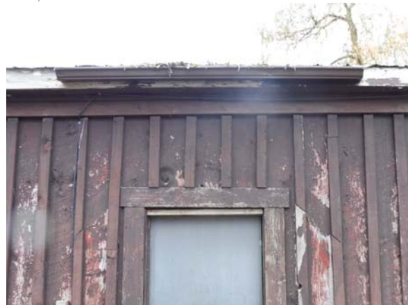
Showing remnant of rain gutter at roofline (ERA, 2017).
