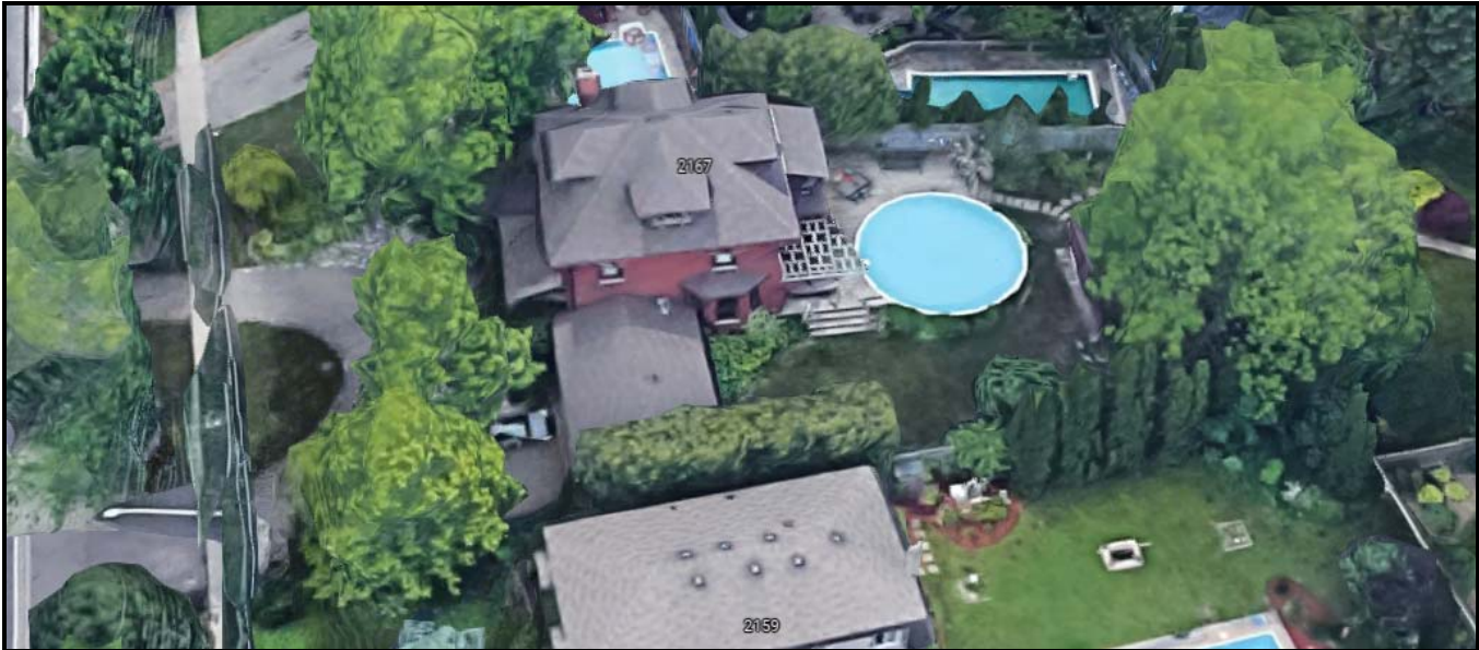
Google aerial showing the overall shape of the house looking west, with a semicircular driveway (backyard has since changed). The four hipped roof dormers are visible. Source: Google
