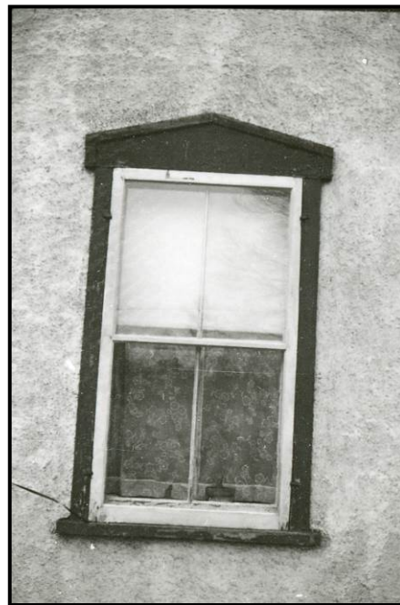
Left: Close up of one of the windows. This one does not have its storm window, but we can see the wooden sash, the pediment, and wooden frame. Source: Planning Services staff photo, 2024.
