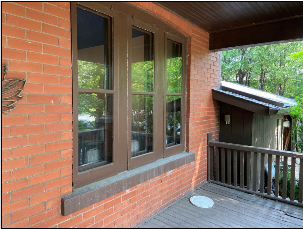
Set of three windows on the east side of the front door. Source: Town of Oakville Planning and Development Staff
