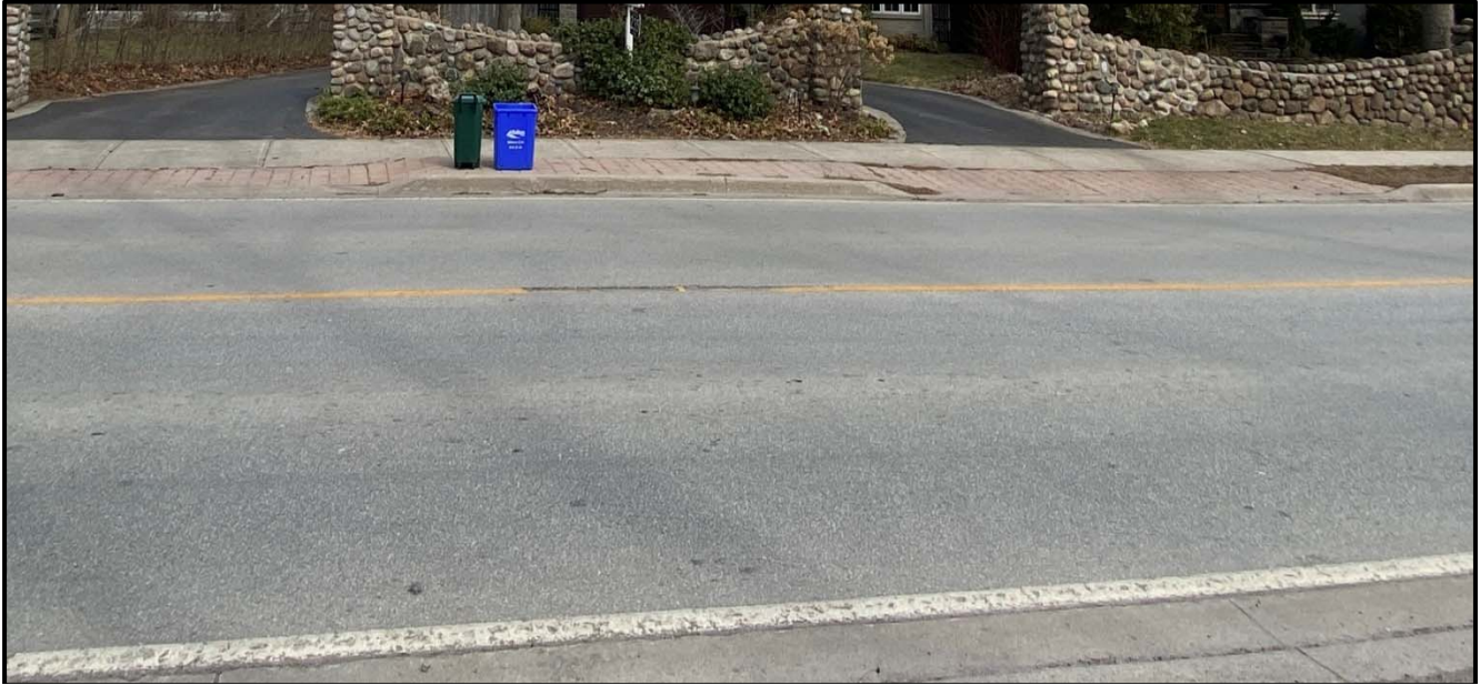
235 Bronte Road, March 2024. Source: Town of Oakville, Planning Services staff photos
