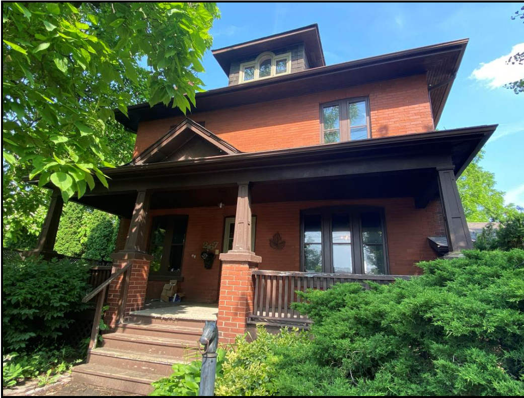
South elevation (front façade).
