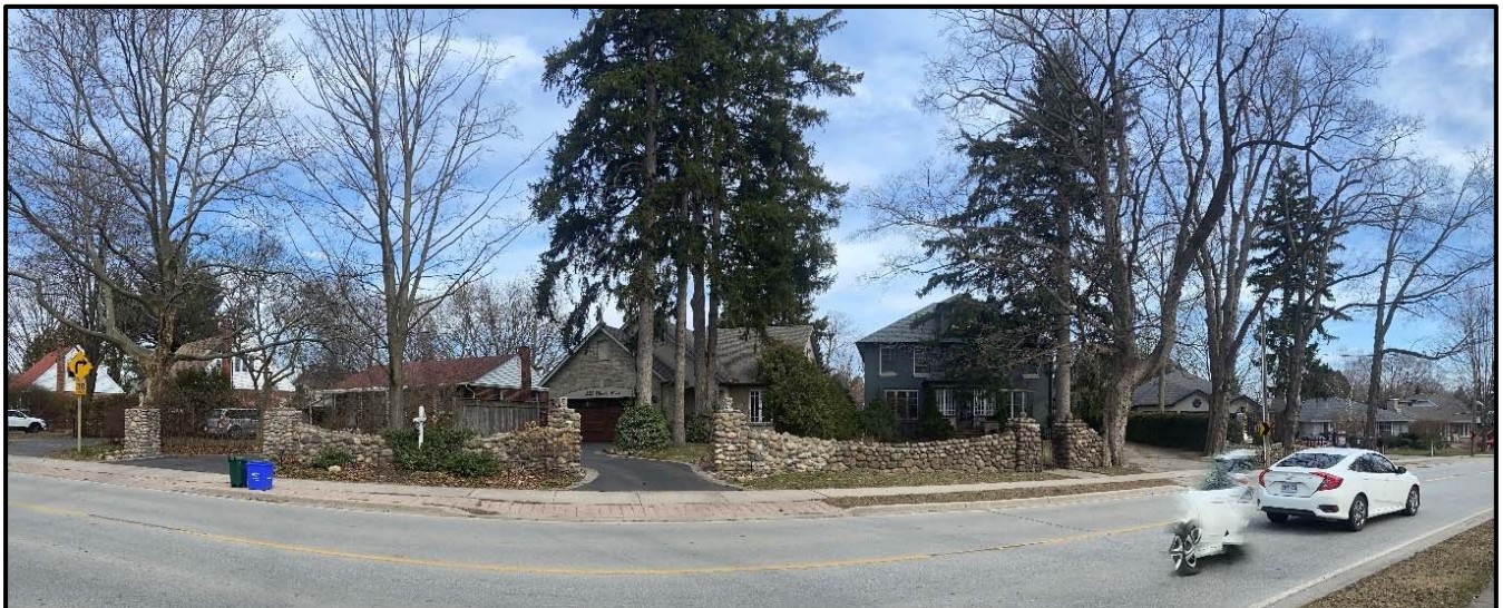
A panoramic view of 225, 231, and 235 Bronte Road showing the extent of the stone wall and pillars. March 2024. Source: Town of Oakville, Planning Services staff photos
