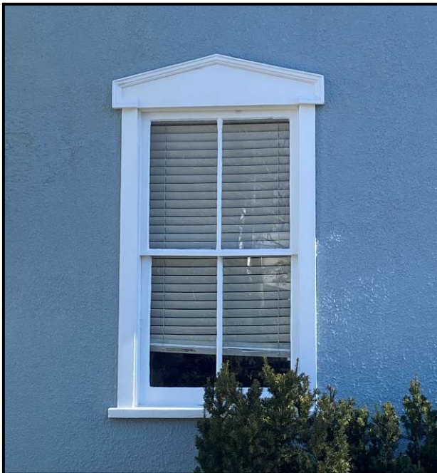
Left: Close up of one of the windows. This one does not have its storm window, but we can see the wooden sash, the pediment, and wooden frame. Source: Planning Services staff photo, 2024.
