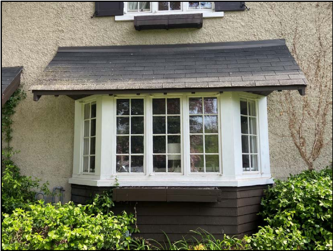
Exposed wooden eaves on the roof over the front bay window on the west elevation, 2024. This is the same on all overhanging rooflines of the house. Source: Town of Oakville Planning Staff
