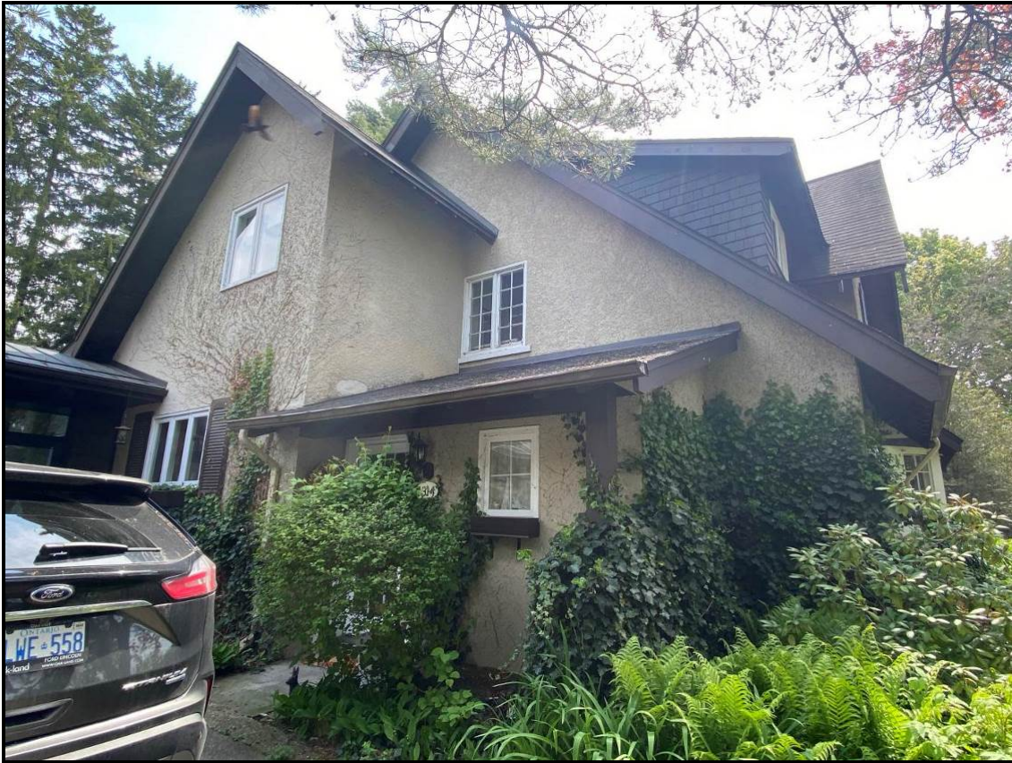
North elevation with 1990s addition on the left, 2024. Source: Town of Oakville Planning Staff
