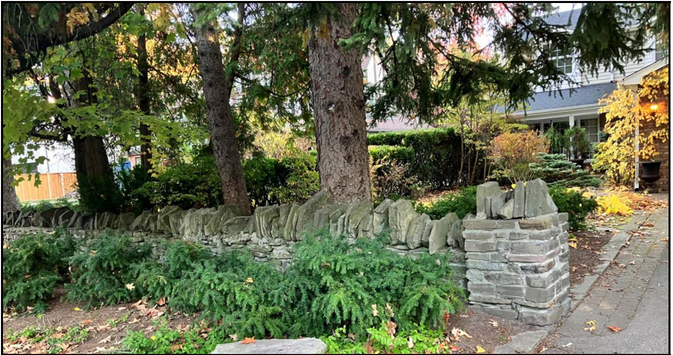
The stone wall in front of 323 Douglas Avenue, 2024. Source: Town of Oakville Planning and Development Staff
