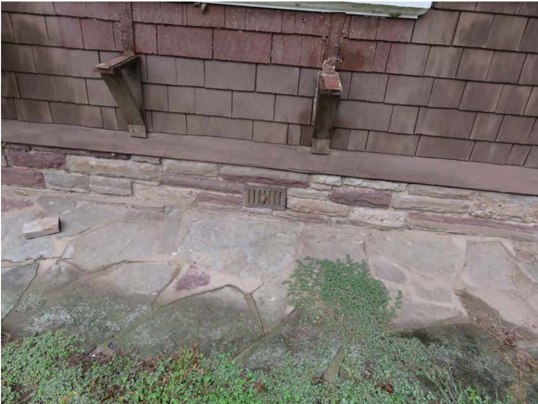
Raised stone foundation – metal grate – brackets for window boxes
