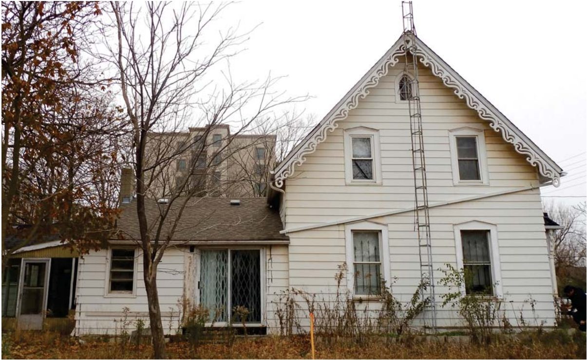
South elevation showing various extensions to the rear of the building (ERA, 2017).
