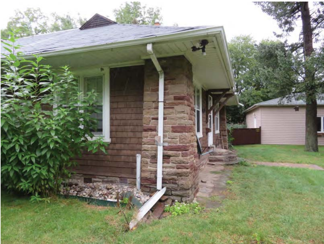
Masonry piers at the corners are flared – wide roof overhang – eyebrow dormers in the low hipped roof
