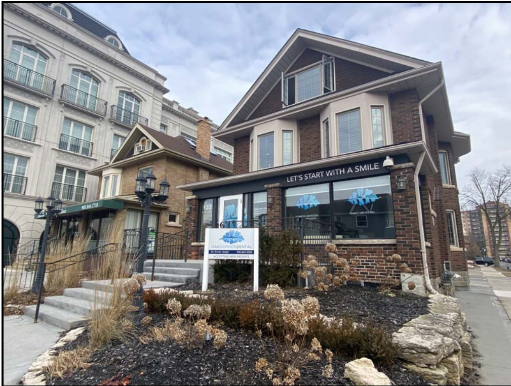
West (front) elevation of the building, 2024. Source: Town of Oakville Planning Services Staff
