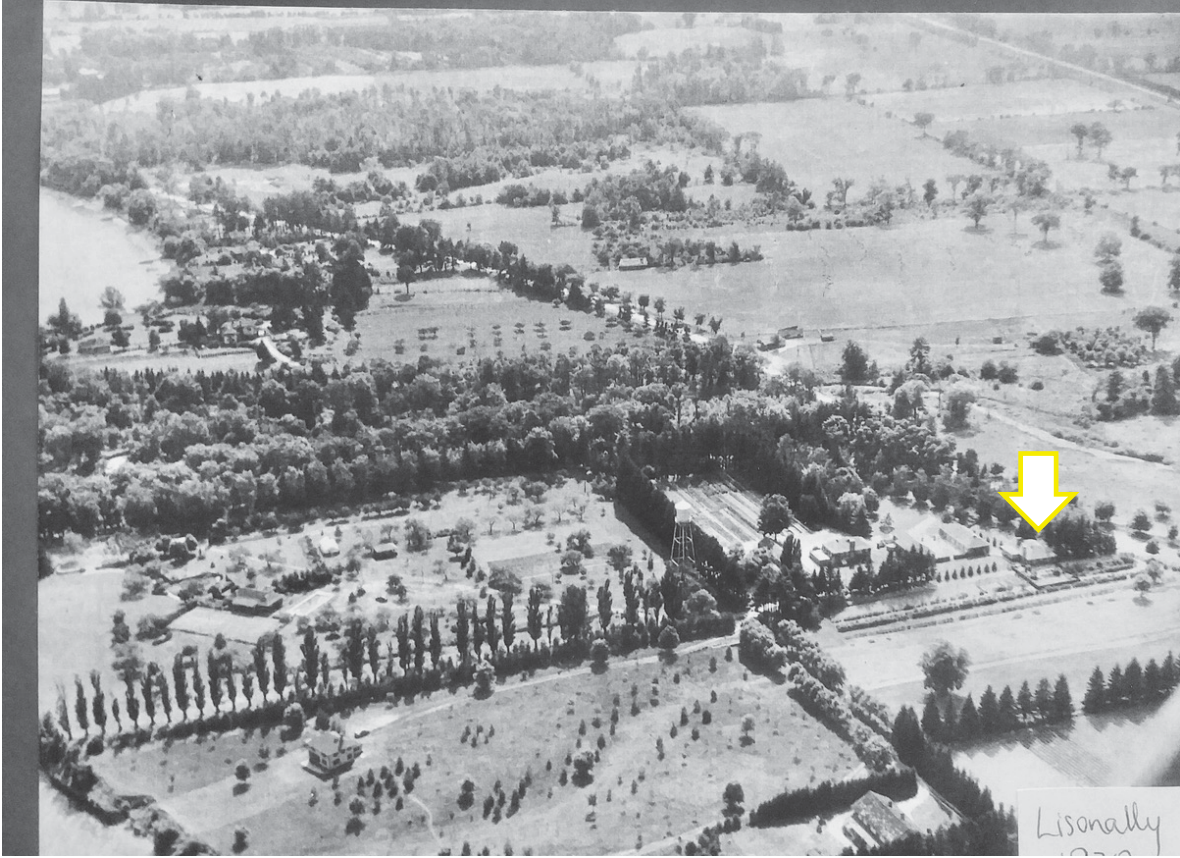
AERIAL VIEW – the Farm Manger’s House is located near the entrance from Lakeshore Road
