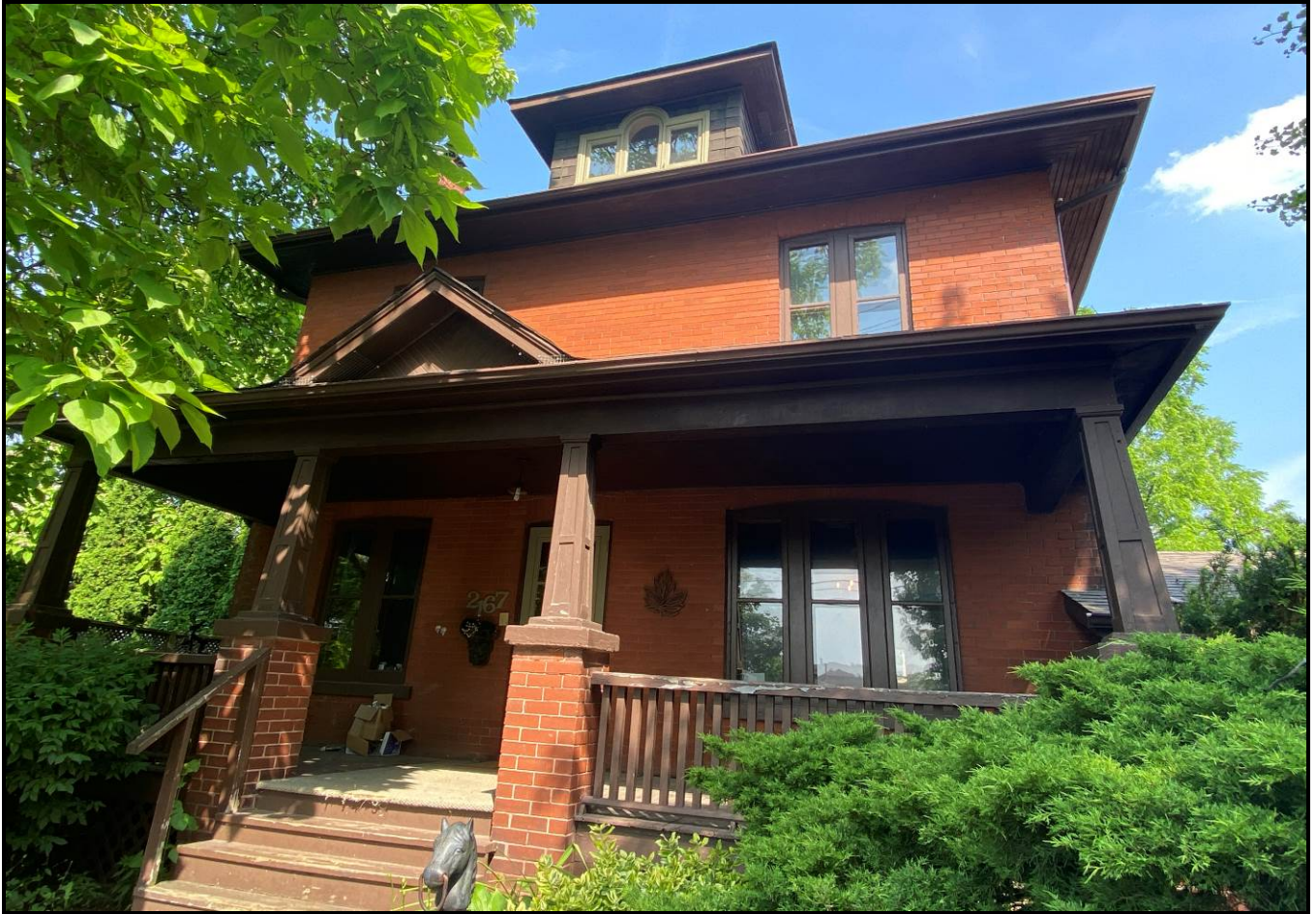
Front elevation of the house, 2024. Town of Oakville Planning and Development Staff
