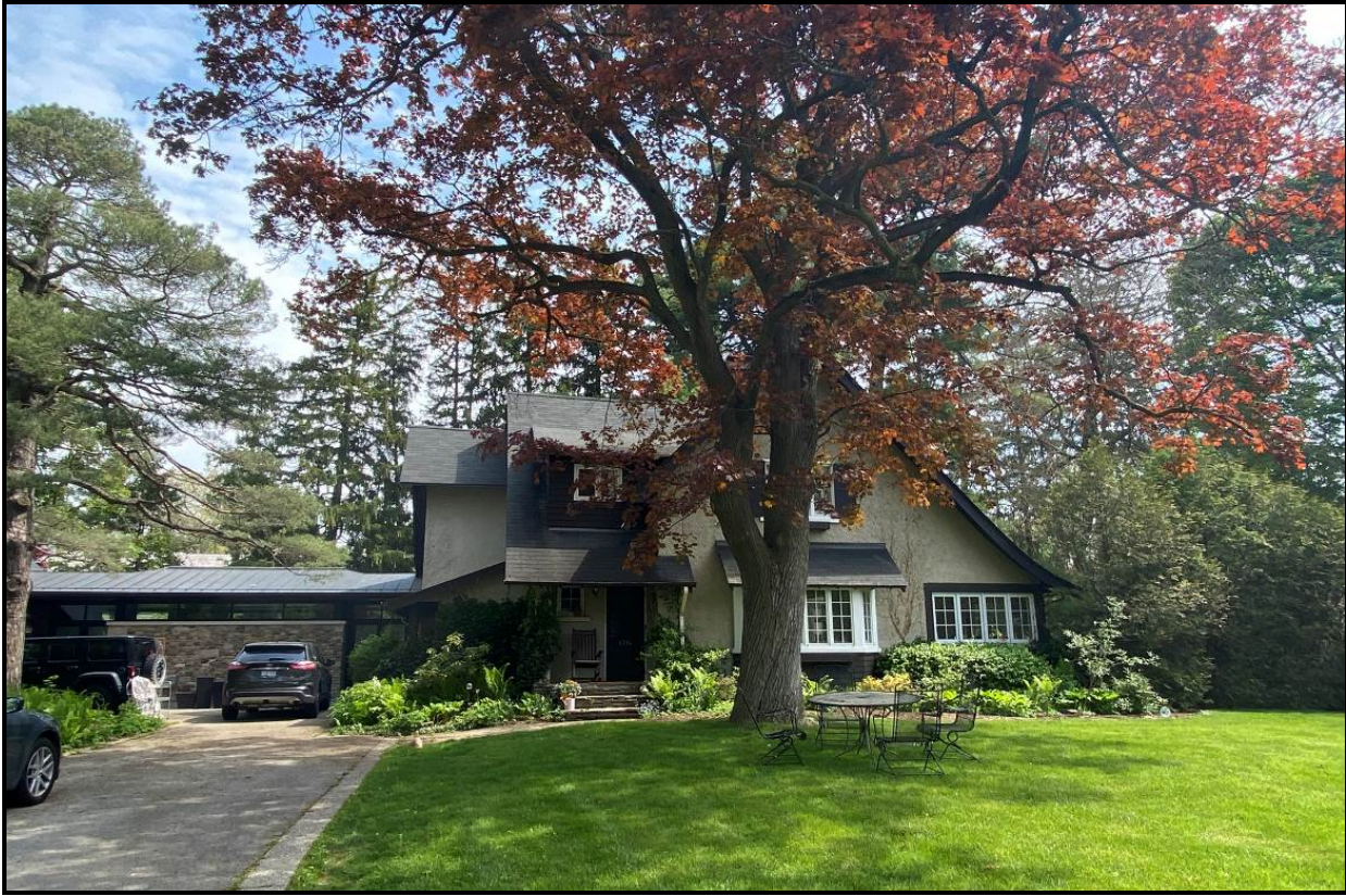
Another view of the west elevation to show the bellcast roofline, 2024. Source: Town of Oakville Planning Services Staff
