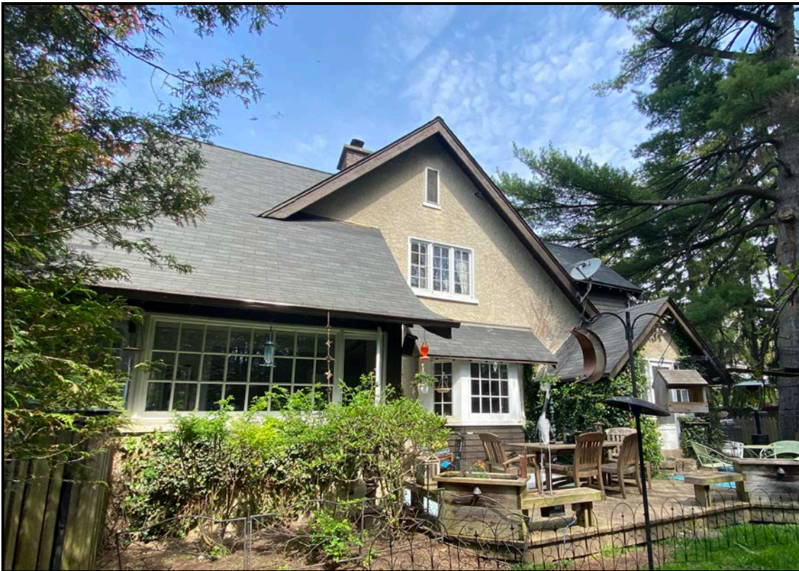
South elevation, 2024. Source: Town of Oakville Planning Staff
