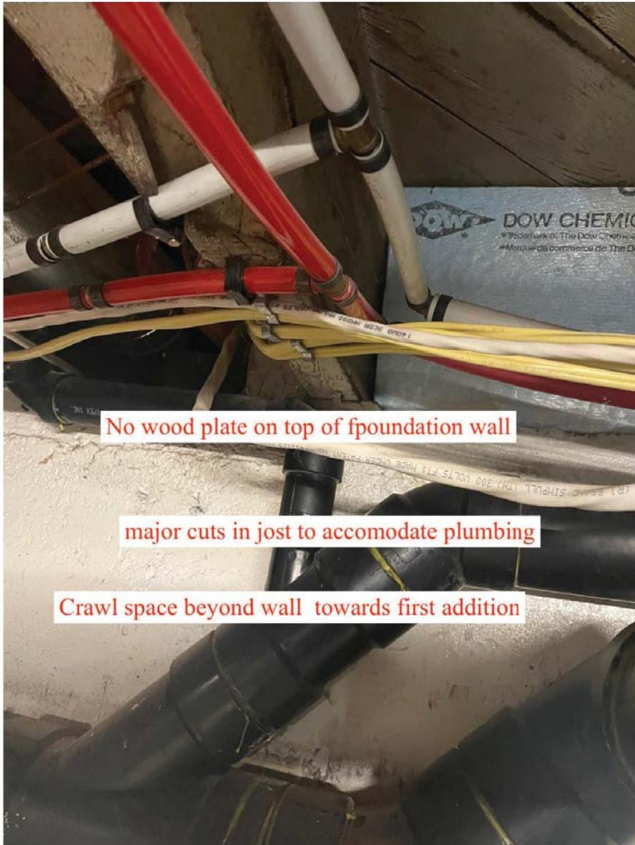
No wood plate on top of foundation wall
