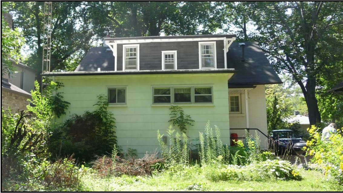
2014 view of the one-storey rear addition built in 1969, before the 2015 renovations. Source: Town of Oakville Planning Services Staff
