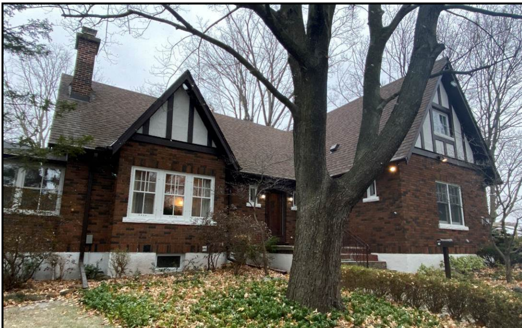
South elevation showing the original front of the house. Town of Oakville Planning Services Staff
