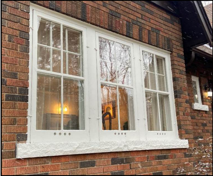
Left: windows on south elevation.
