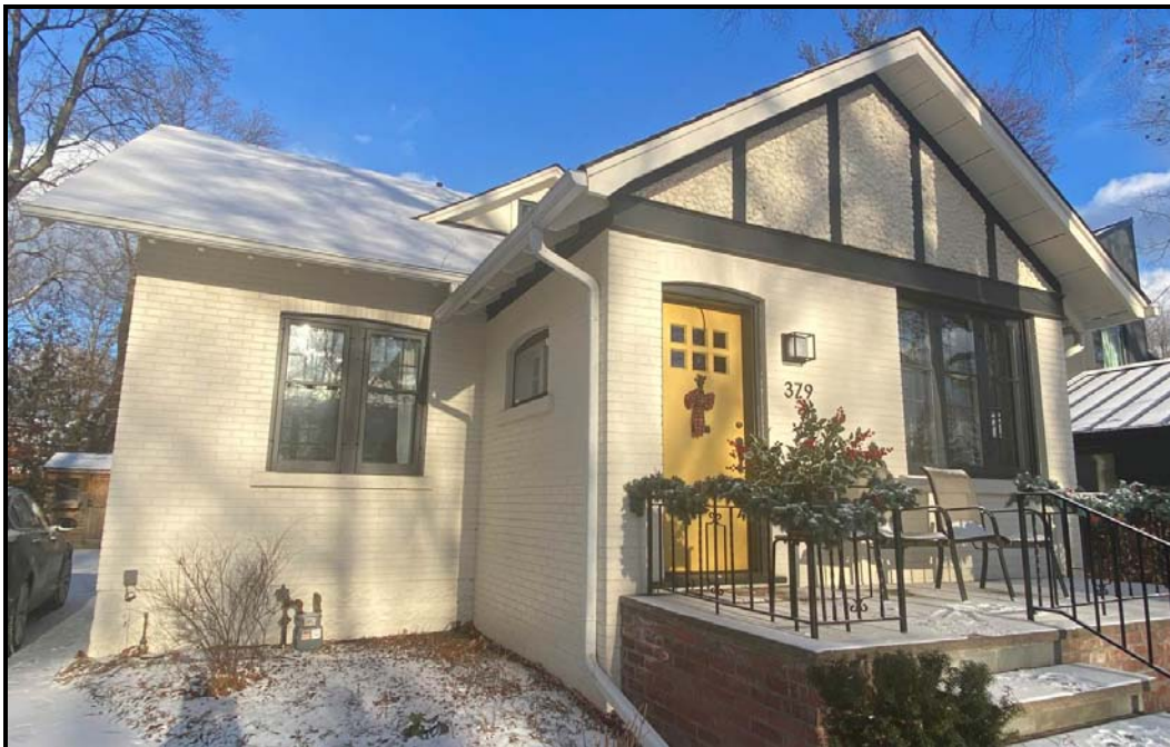
West façade of the house, 2024. Source: Town of Oakville Planning Services Staff
