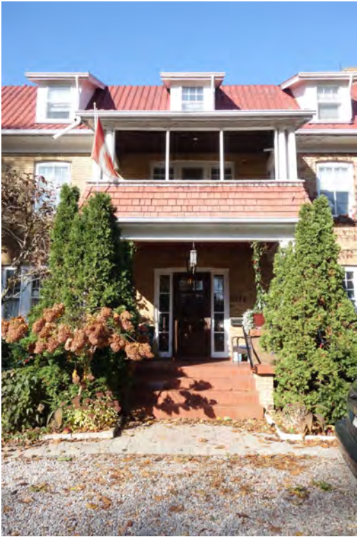
3171 LAKESHORE ROAD W: Front porch
