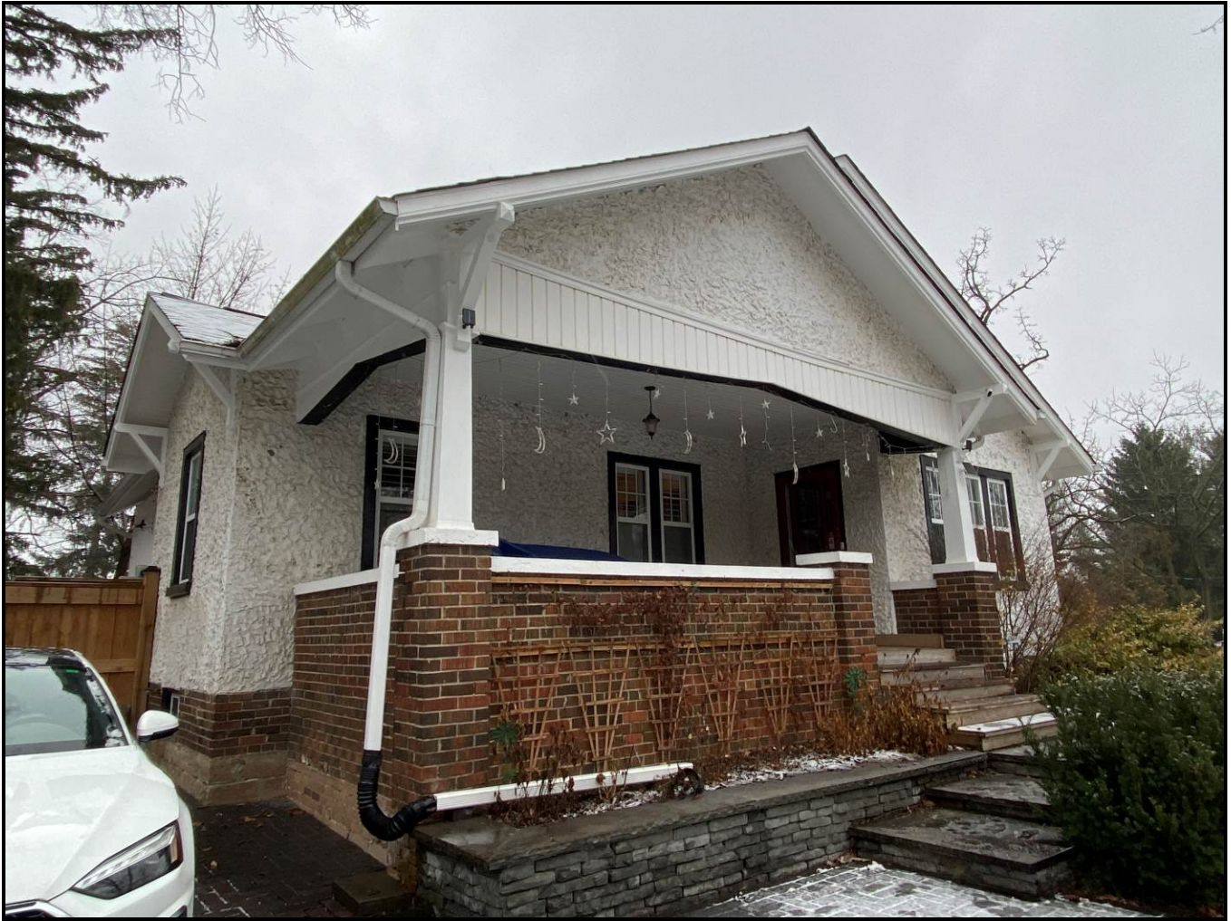
West elevation of the house, 2024. Source: Town of Oakville Planning Services Staff
