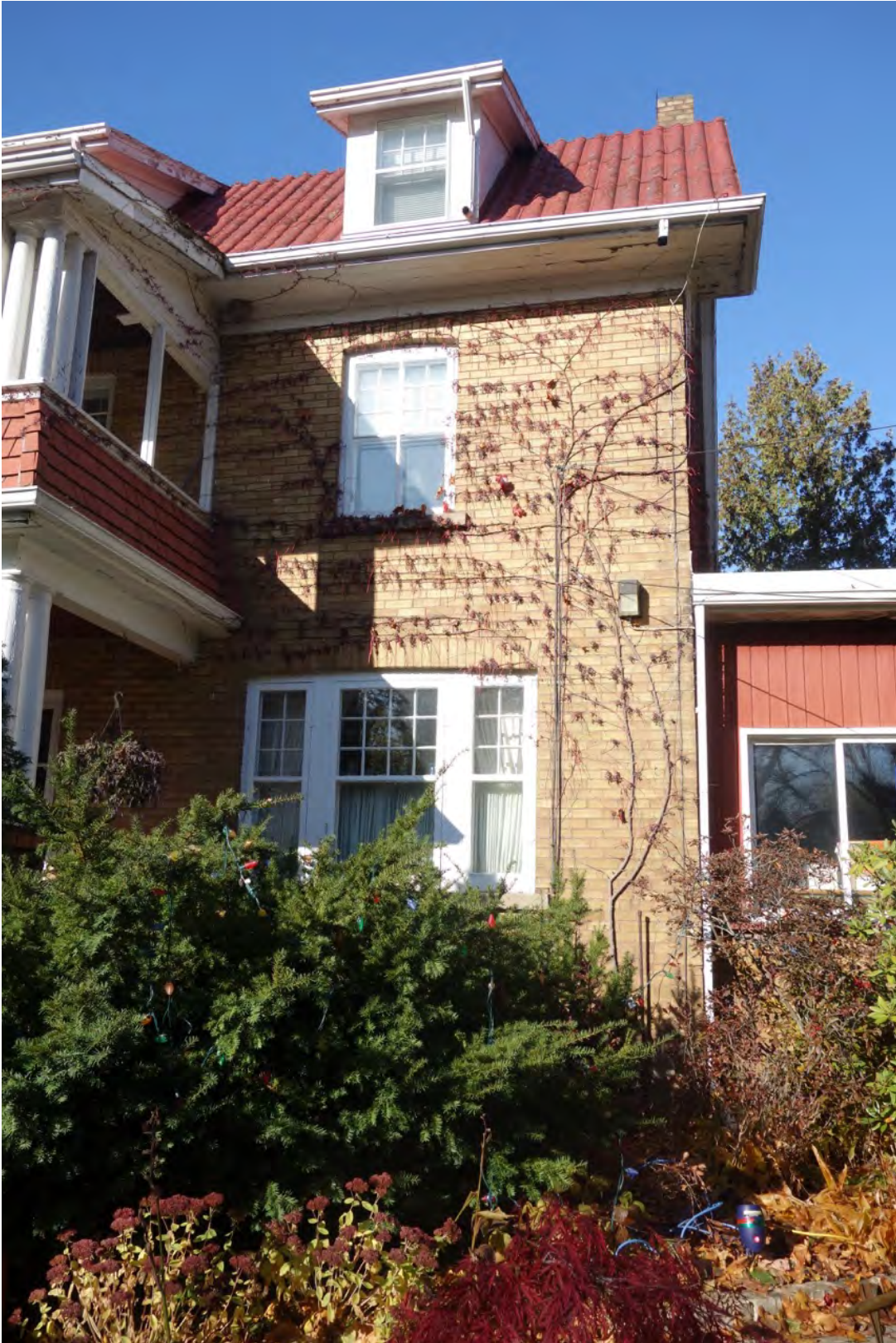
3171 LAKESHORE ROAD W: Front elevation – buff brick – 12 over 1 windows
