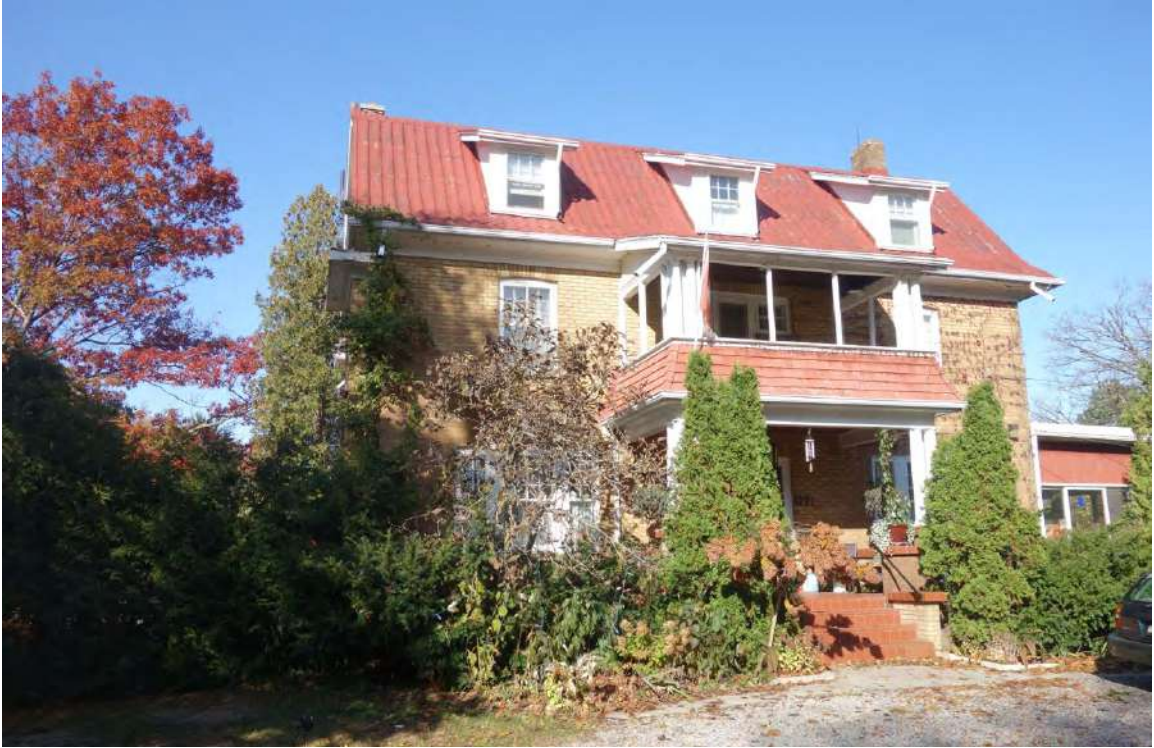
3171 LAKESHORE ROAD W: Main elevation
