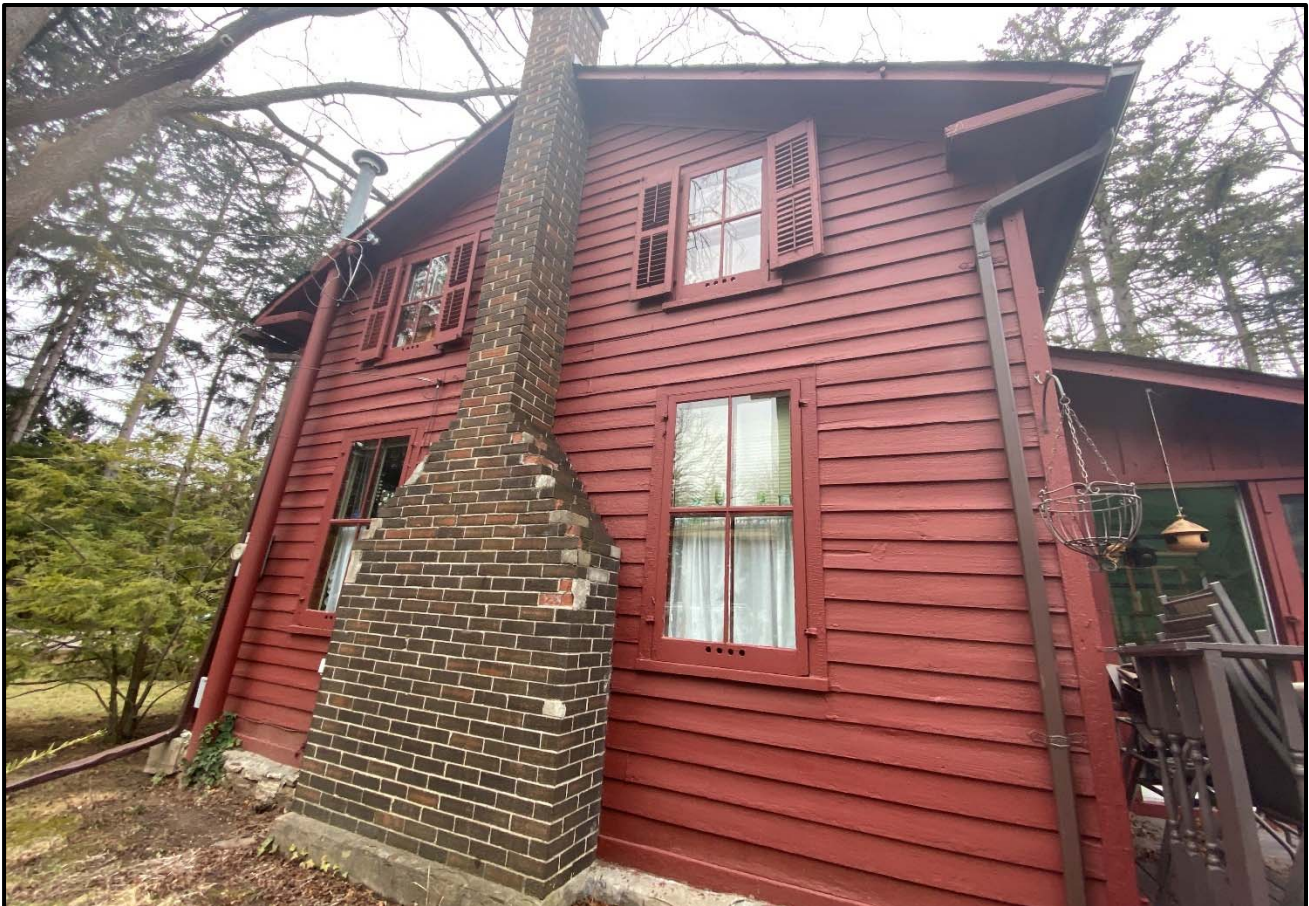
The south elevation of the original portion of the house. January 2024, Source: Town of Oakville Planning Services staff photo of Historic Buildings
