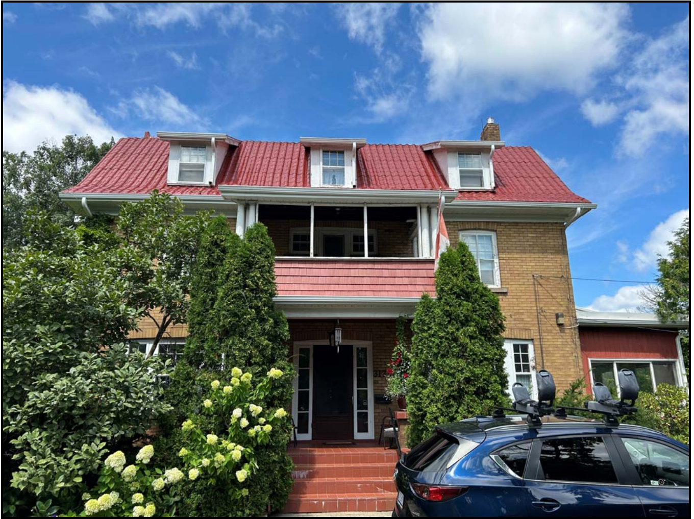
View of the front porch, showing the shingled side and columns, with the front door visible. Source: Town of Oakville Planning Services Staff
