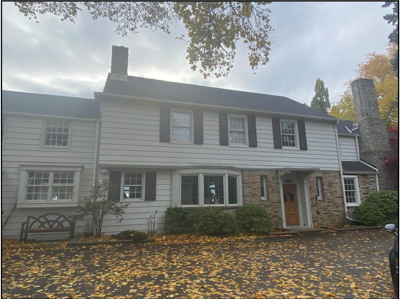
North elevation showing stone veneer on one side and not the other. Also note the small stone-clad bump out beside the chimney. Source: Town of Oakville Planning Services Staff
