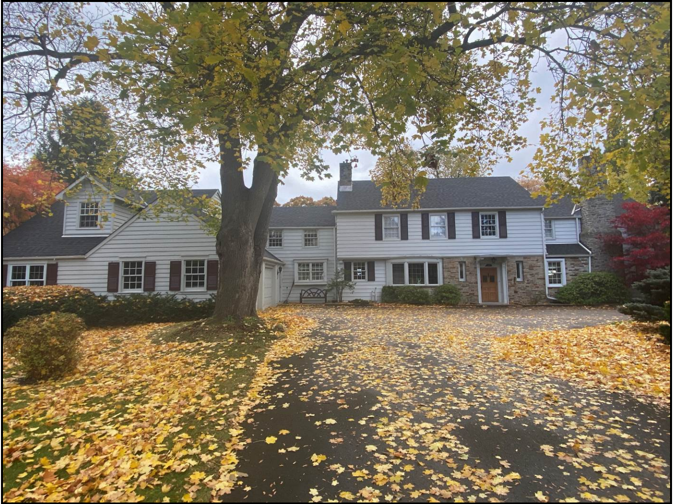
North elevation of the property, 2023. Source: Town of Oakville Planning Services Staff
