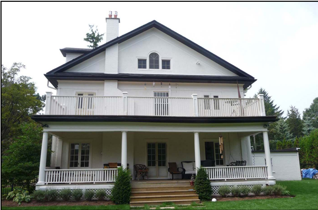
Open porch in 2010. Source: Town of Oakville Planning Services Staff
