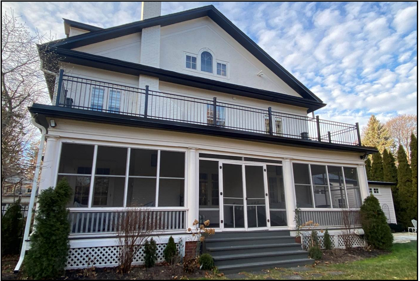
East elevation, 2023. Source: Town of Oakville Planning Services Staff
