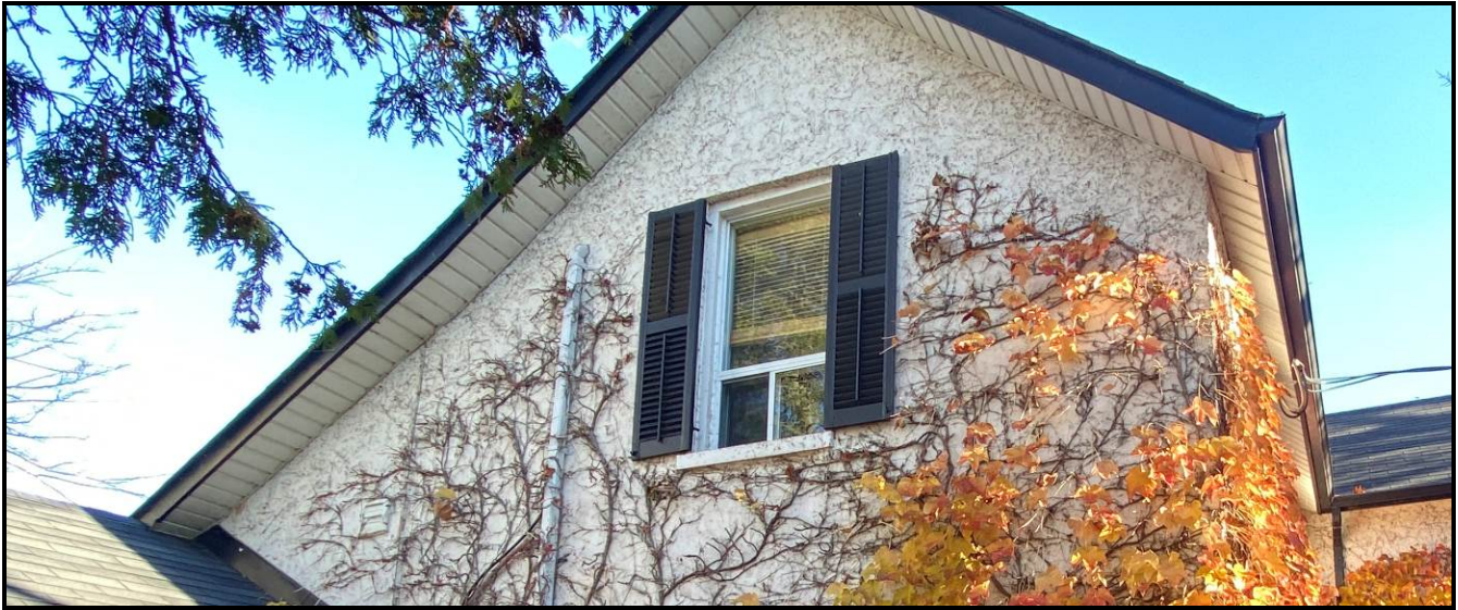
North elevation stucco, showing a pebbled appearance. It is similar to the stucco on the one-storey portion. Source: Town of Oakville Planning Services Staff
