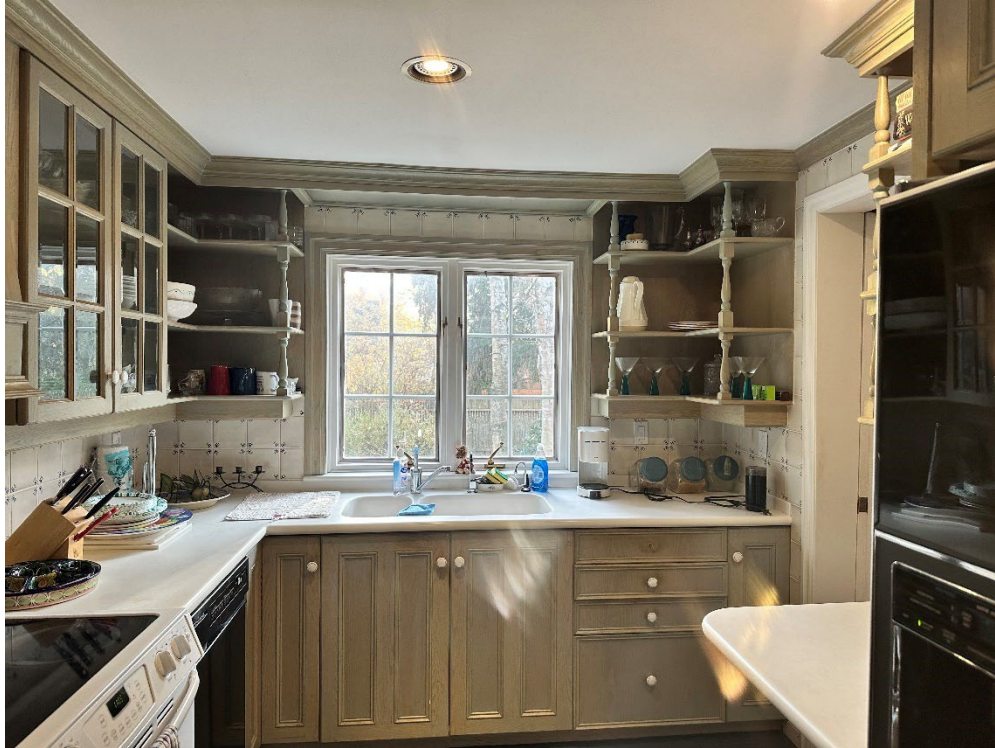
KITCHEN "A". NOTE INTERIOR FINISHES NOT ORIGINAL
