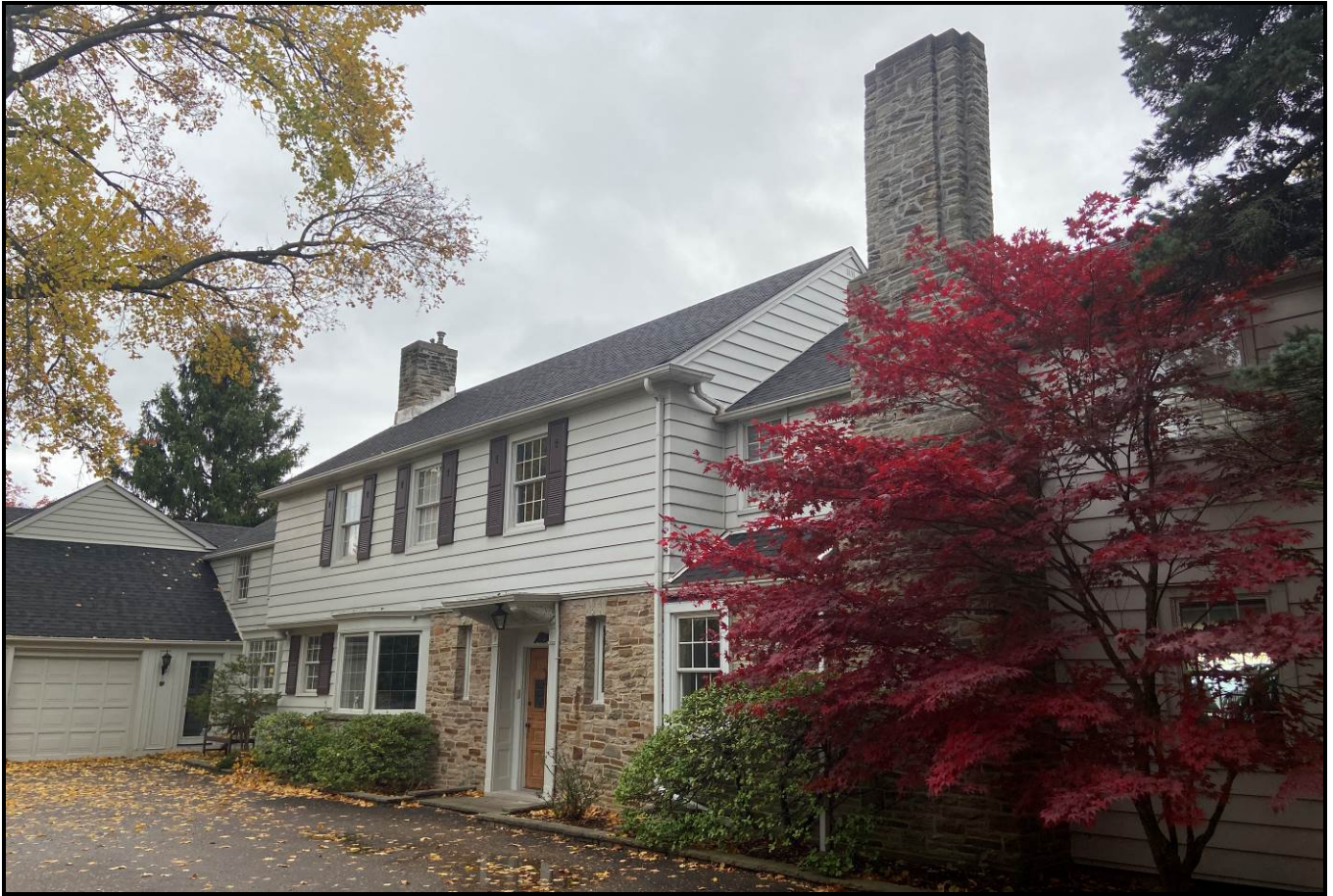
North elevation showing two chimneys. Source: Town of Oakville Planning Services Staff
