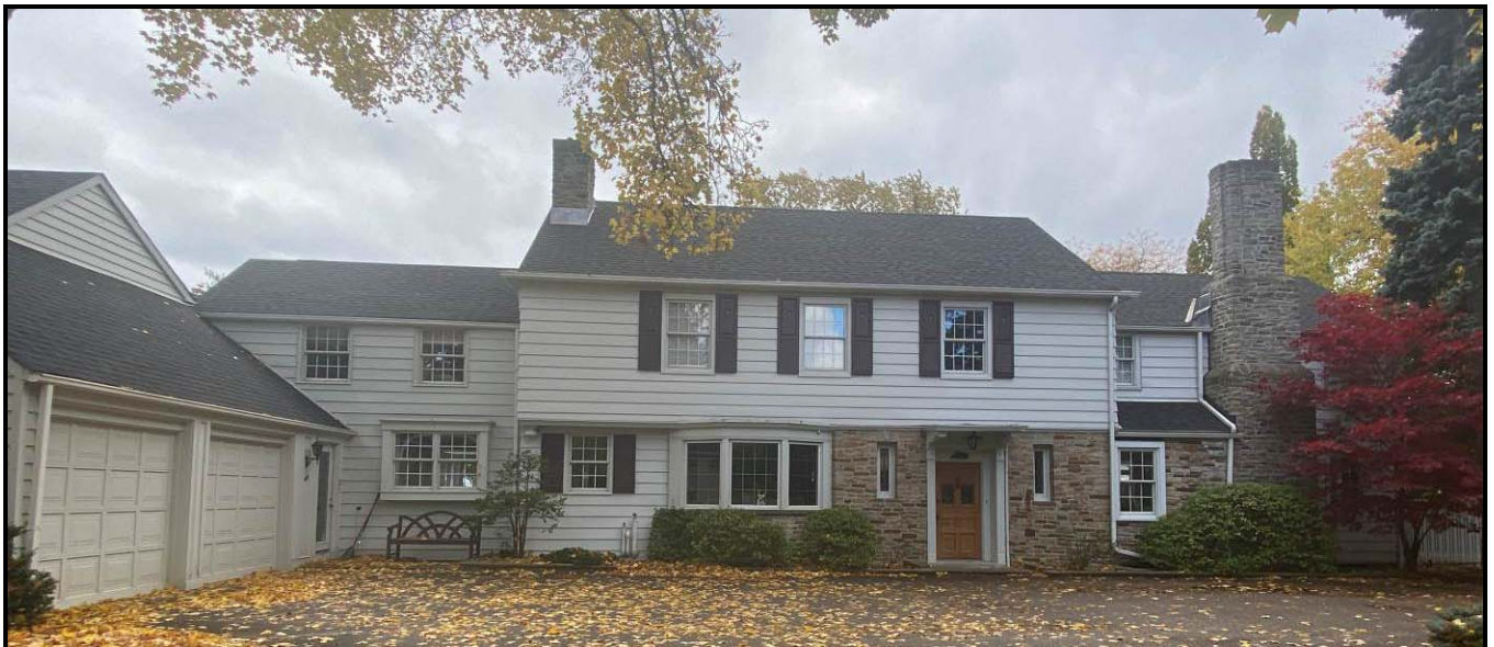
Fenestration on the north elevation.
