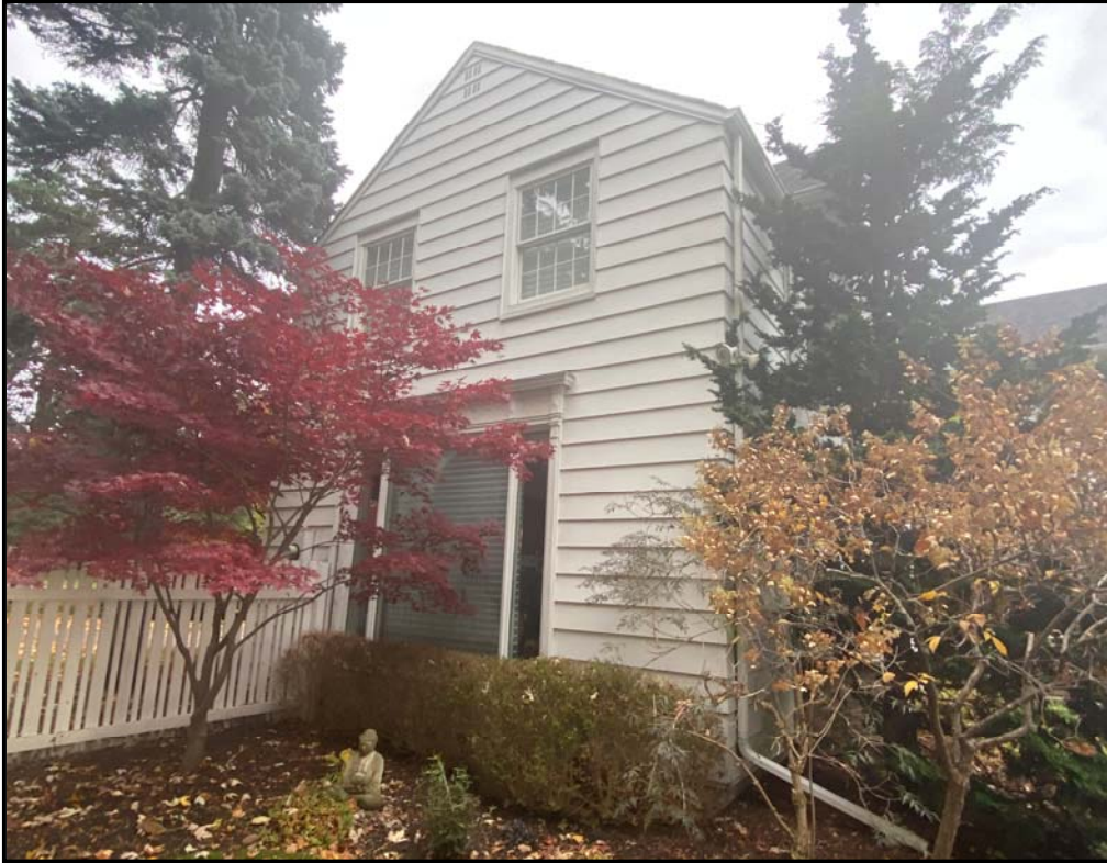
Large window on first storey of west elevation. Source: Town of Oakville Planning Services Staff
