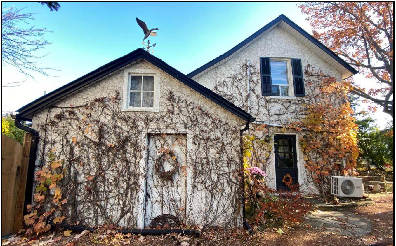
North elevation showing the two entrances. Source: Town of Oakville Planning Services Staff
