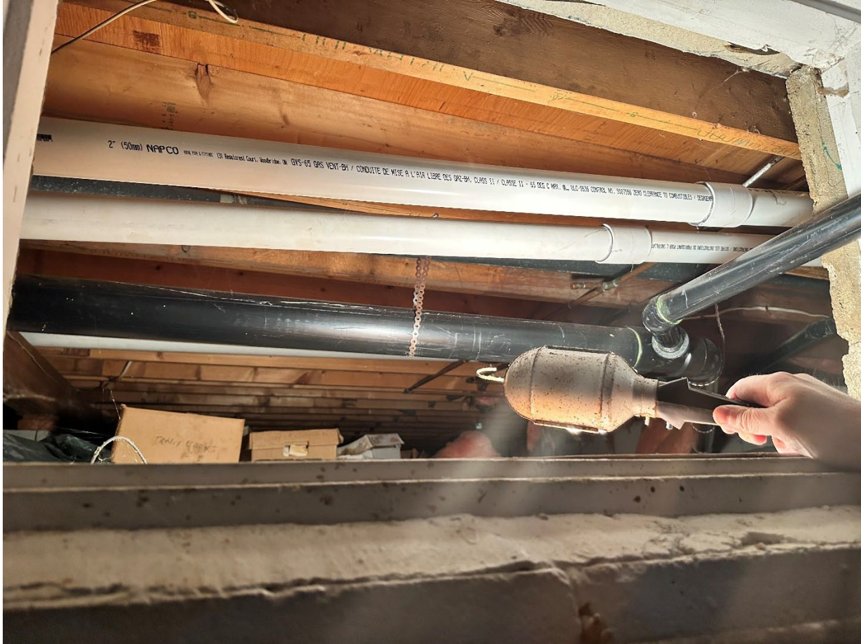
CRAWLSPACE UNDER "B" SHOWING MODERN FRAMING MATERIALS
