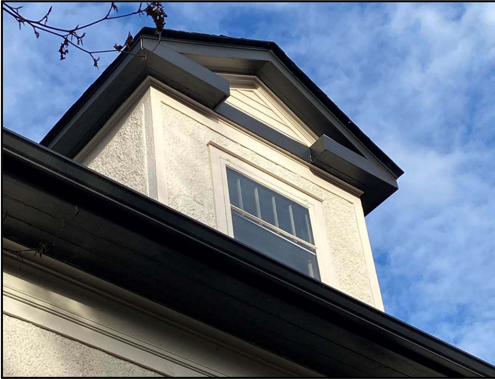
Close-up of one of the dormers, which also shows the stucco and timber edging. Source: Town of Oakville Planning Services Staff
