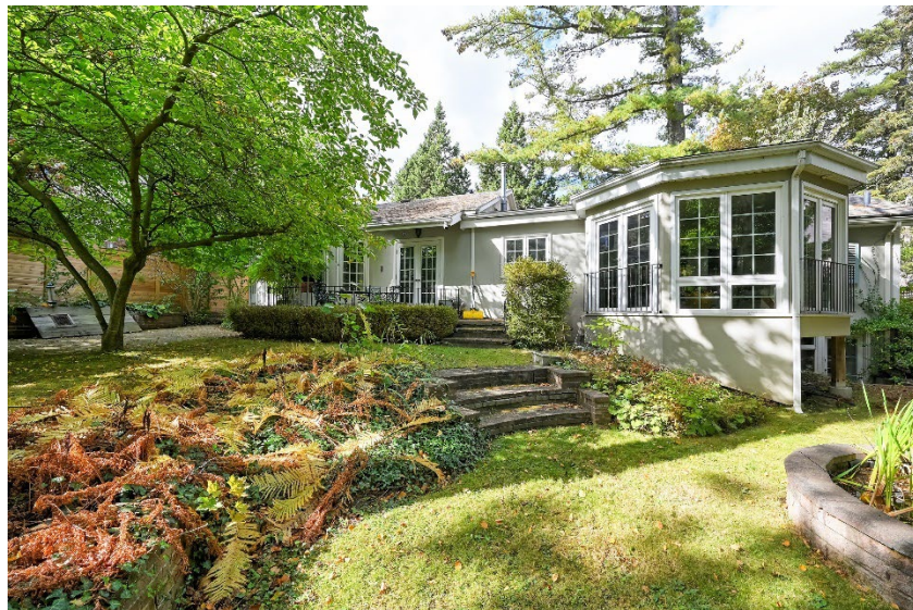
FRONT AND REAR ELEVATIONS SHOWING REGULAR MAINTENANCE, SERVICEABLE CONDITIONS
