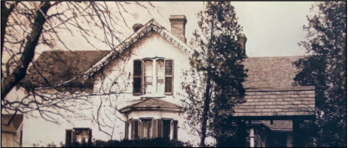
Bargeboard on the west elevation. The three chimneys are also visible. Source: Town of Oakville Planning Services Staff
