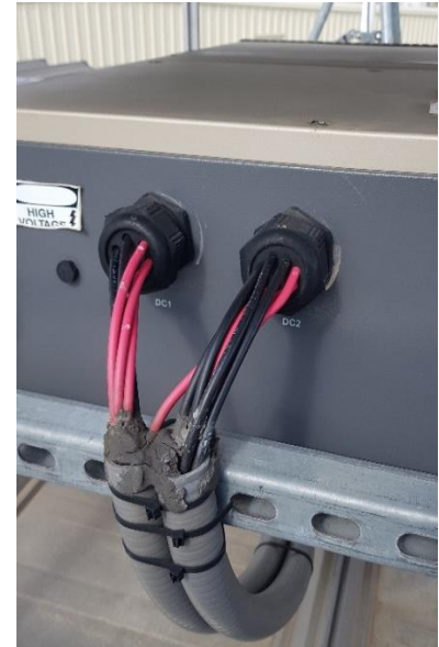
Picture 11: Home-run Wiring
