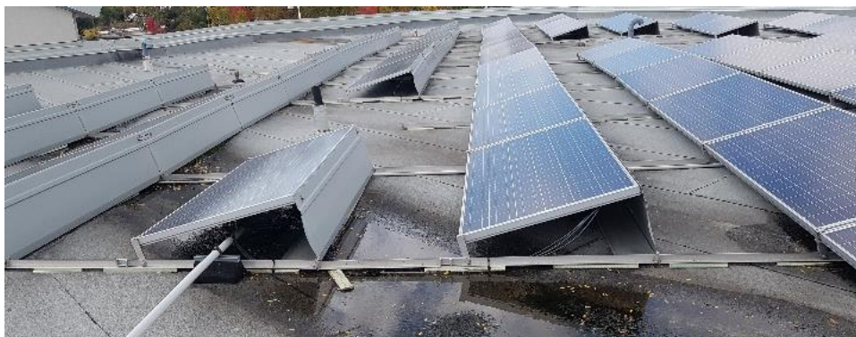
Picture 14: Hanging PV Wire
