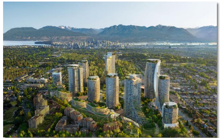
Photograph 19: Oakridge Centre Redevelopment in Vancouver
