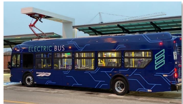
Photograph 25: Brampton Transit Electric Bus Charging
